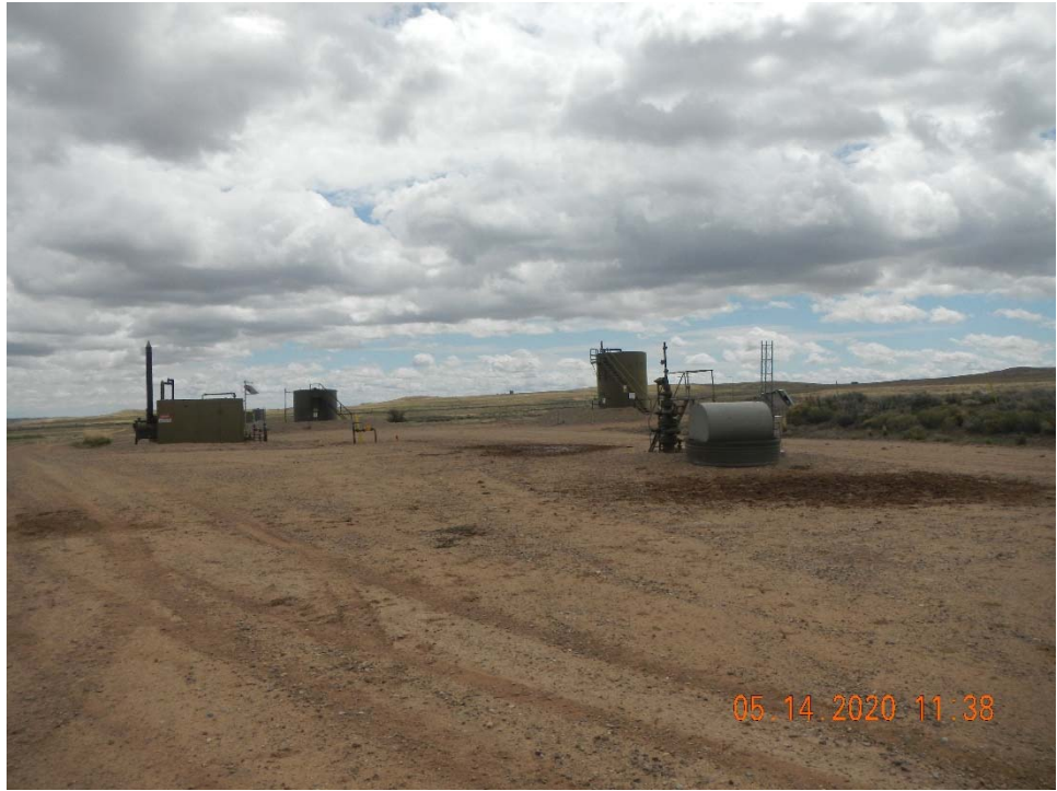
Photo 1. Overview of location taken facing southeast.
