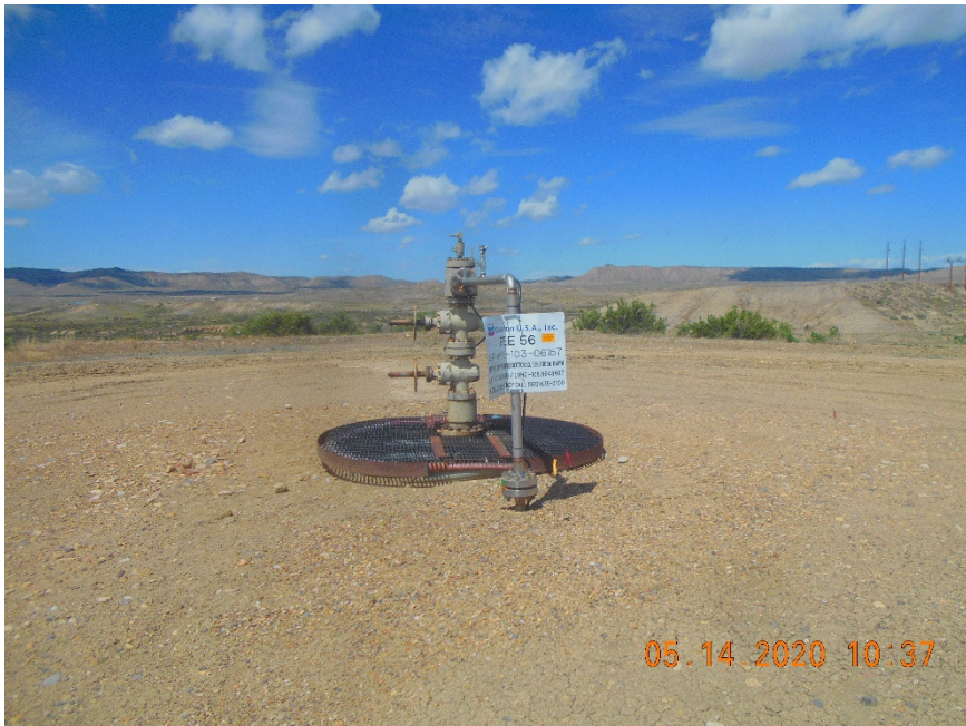
Injection wellhead
