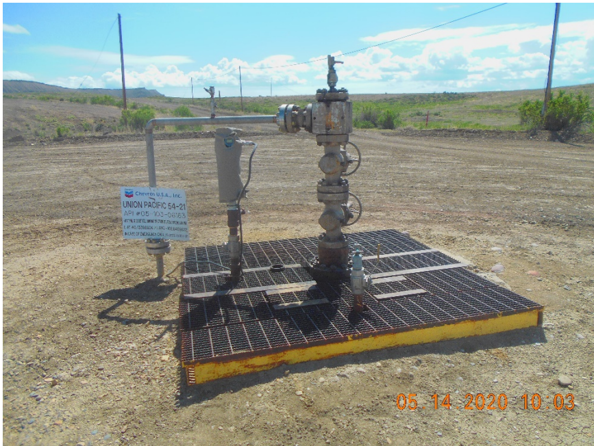
Injection wellhead
