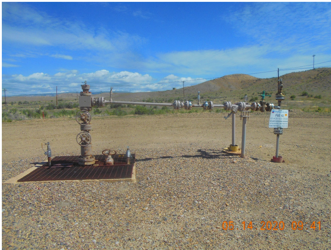
Injection wellhead- Temporarily Abandoned
