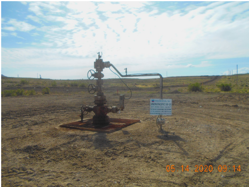
Injection wellhead
