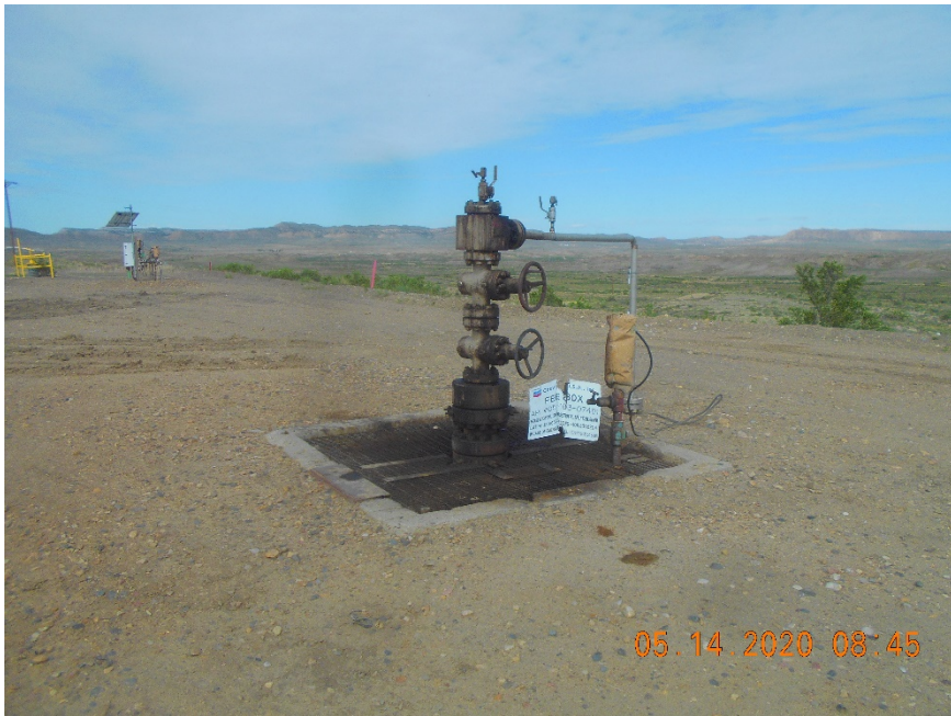
Injection wellhead
