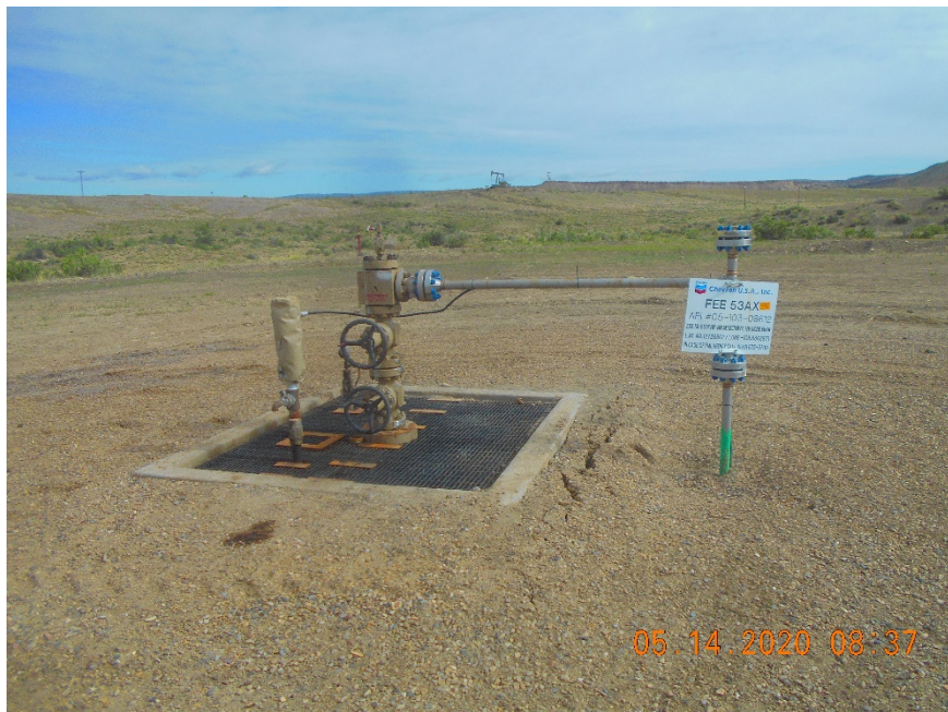
Injection wellhead
