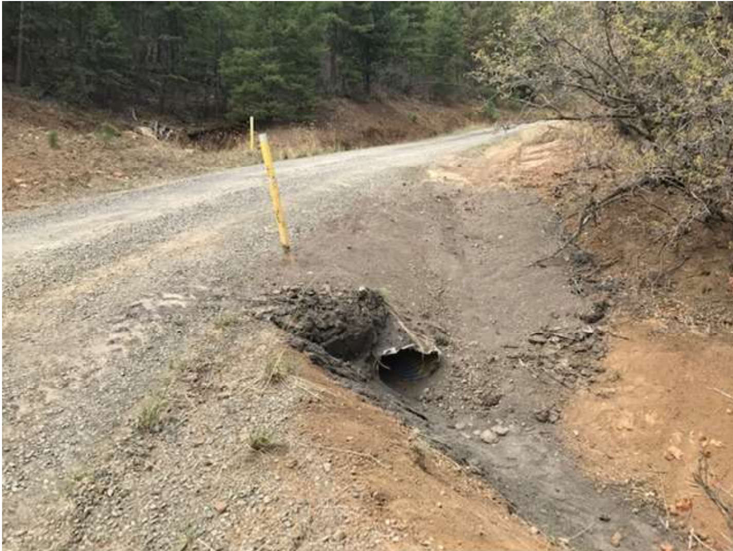
PHOTO 3: THE EROSION ON THE CULVERT OUTLET WAS BACKFILLED.
