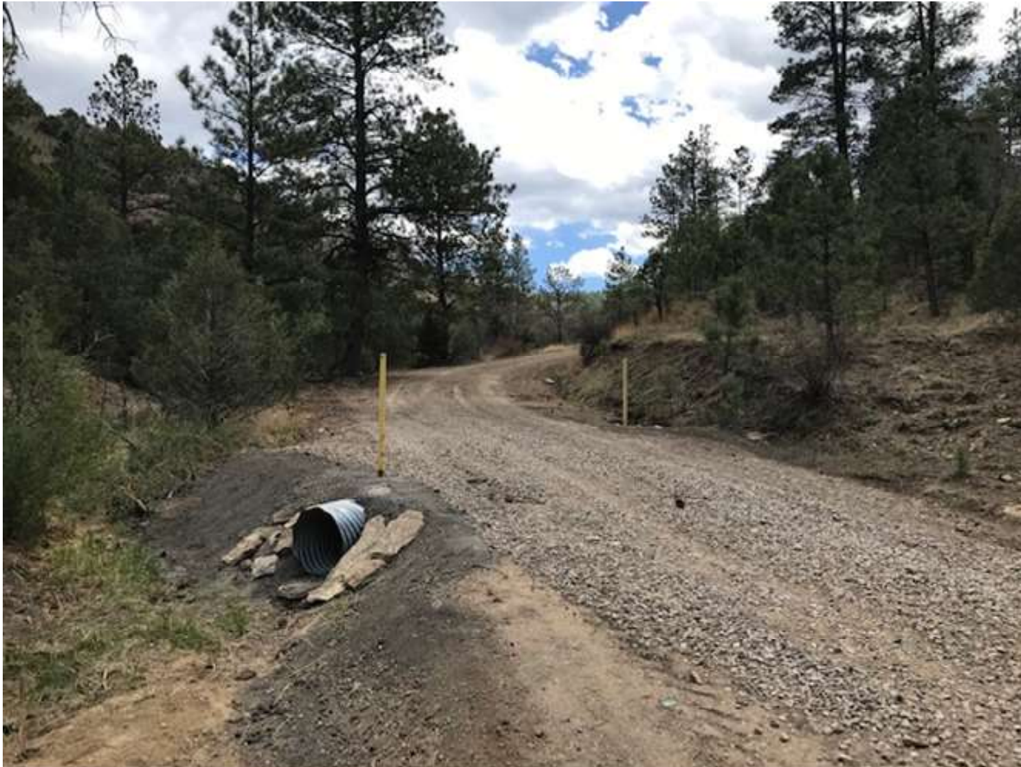
PHOTO 4: AN ADDITIONAL CULVERT WAS INSTALLED ON THE MAIN LEASE ROAD IN BIG BINGHAM CANYON.
