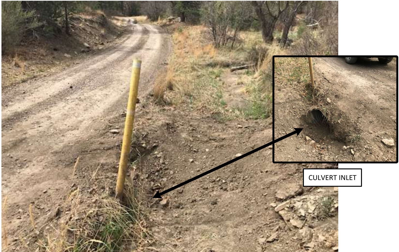
PHOTO 1: FACING SOUTHEAST ALONG THE MAIN LEASE ROAD IN LITTLE BINGHAM CANYON. THE SEDIMENT ACCUMULATION WAS REMOVED FROM THE CULVERT INLET.
