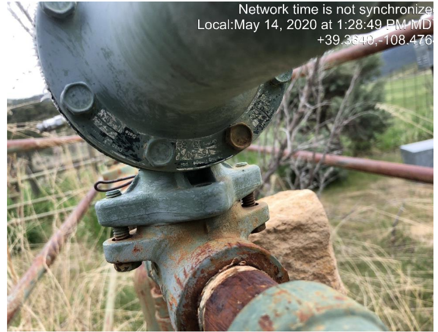
Photo #1193 Little joe regulator pressure plate.
