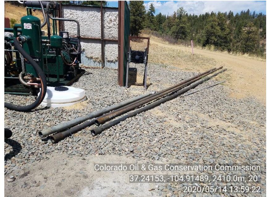
PHOTO 4: UNUSED EQUIPMENT LEFT ON LOCATION (JTS OF TBG BUMP & STATER). REMOVE UNUSED EQUIPMENT COMPLY WITH RULE 603.f. 8-14-20.
