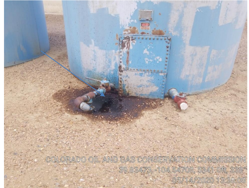
Pic 6 mechanical issue with tank/stained soil
