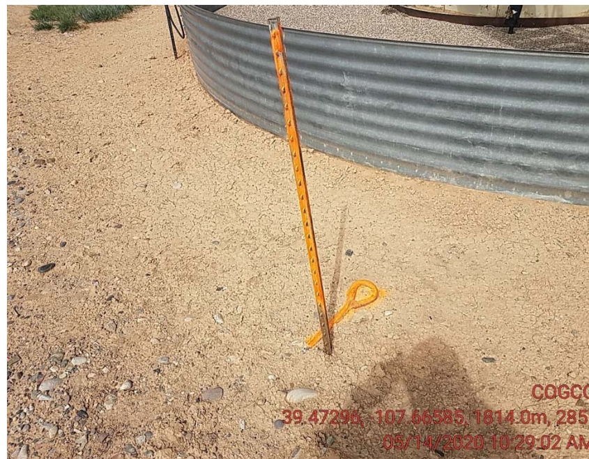
follow up inspection
