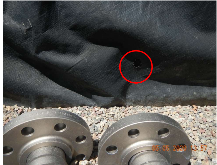
Hole in tank battery secondary containment liner
