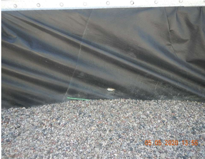
Hole in tank battery secondary containment liner
