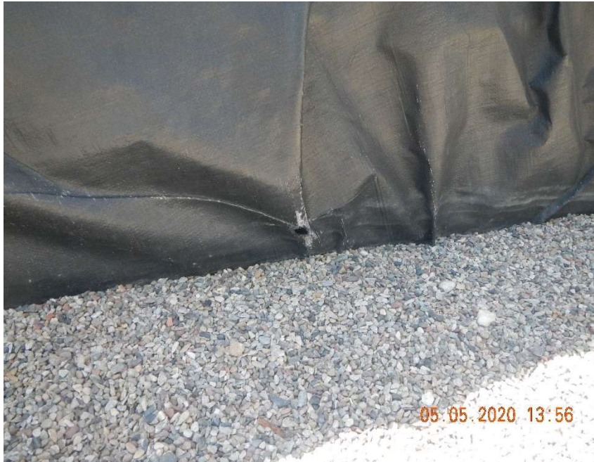
Hole in tank battery secondary containment liner
