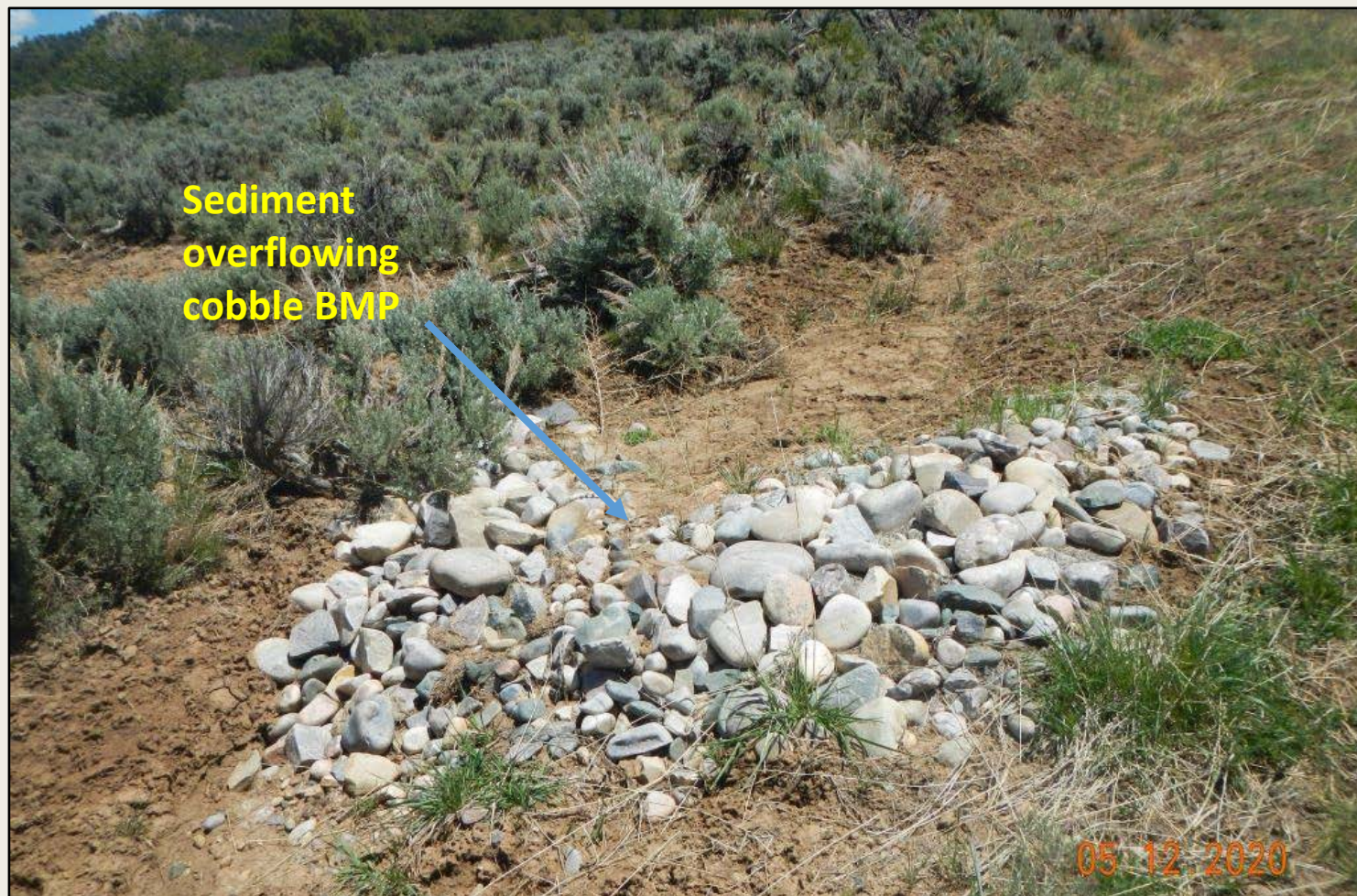
Photo 4. View of stormwater BMP in the northern project area, that is full of sediment.
