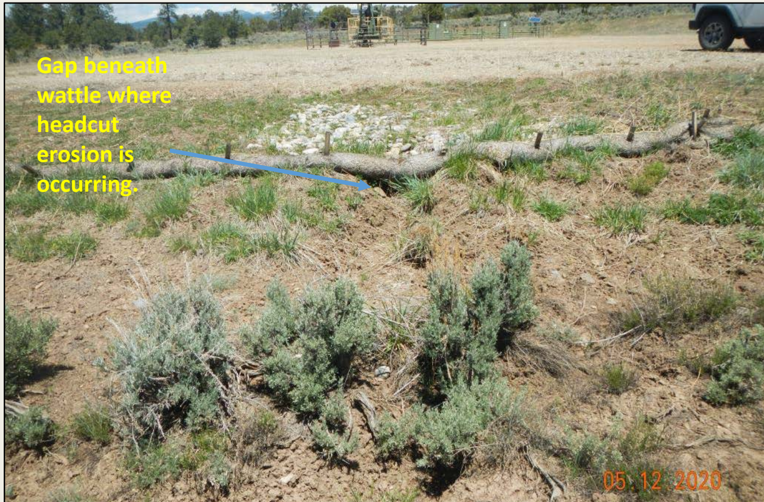
Photo 5. View of wattle and cobble BMPs in the southern project area. Large gap and headcut present beneath the wattle. Improved BMPs are needed here.
