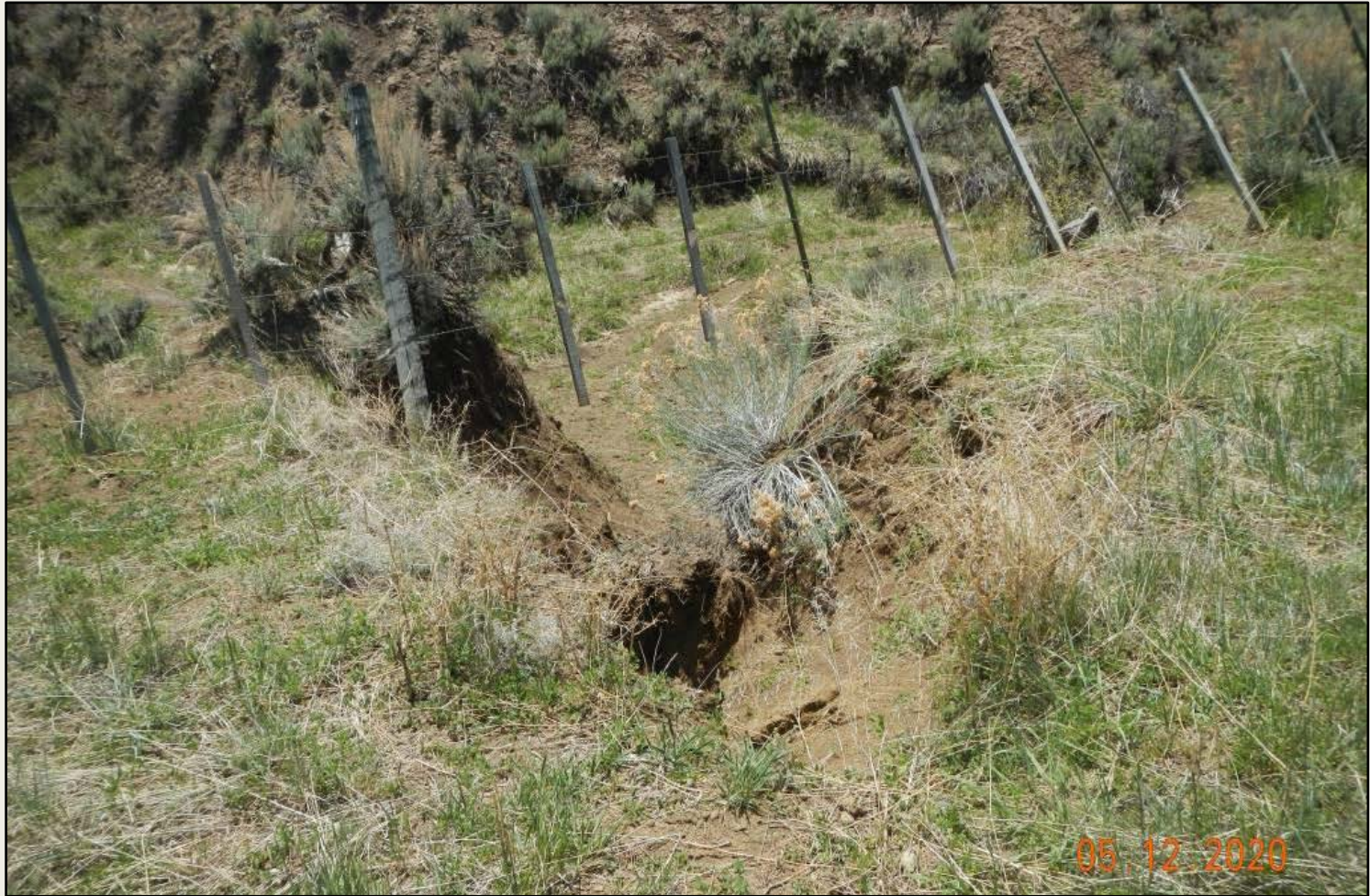
Photo 4. View of erosional head-cut in Photo 3, facing downstream. Stabilization is needed here.
