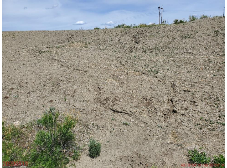
Photo 6: Photo taken from the southeast end of the Location. Photo shows erosion degradation due to stormwater runoff from the Location is evident.
