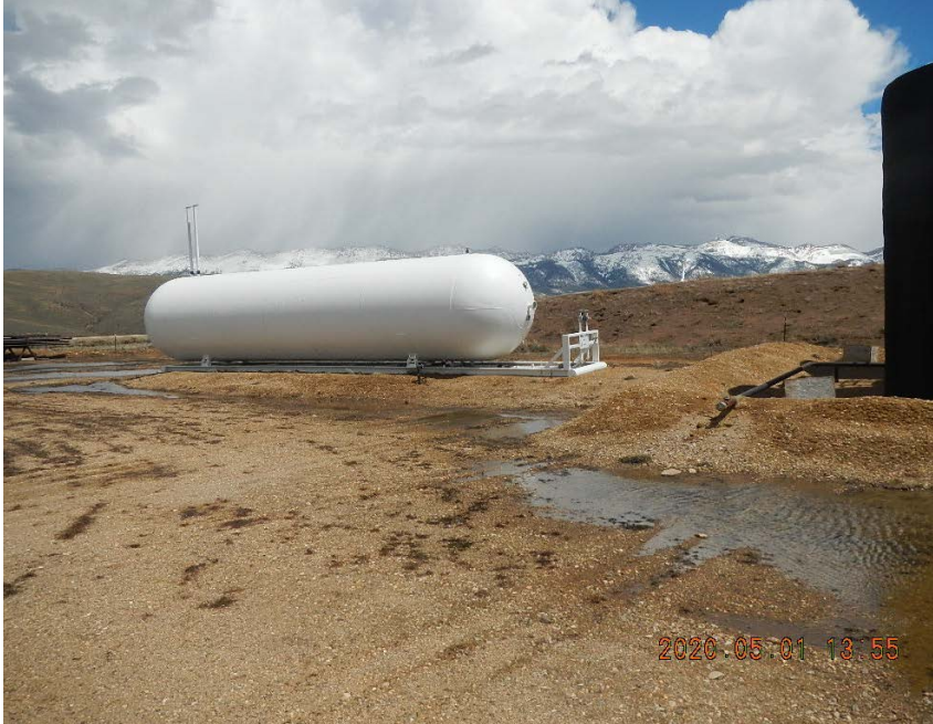
Propane tank not labeled or placard.
