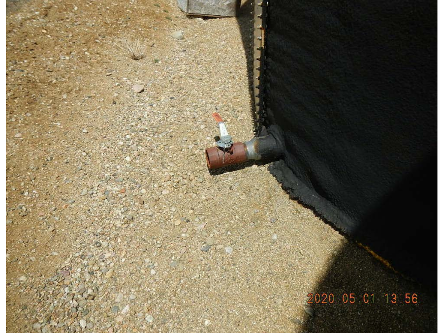
Valve with handle not blind plugged. Note: There was evidence of livestock accessing Facility.
