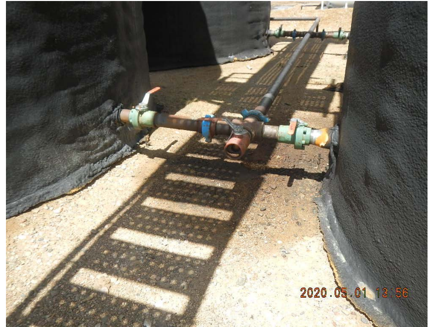
Tank 0030, staining beneath hammer unions.
