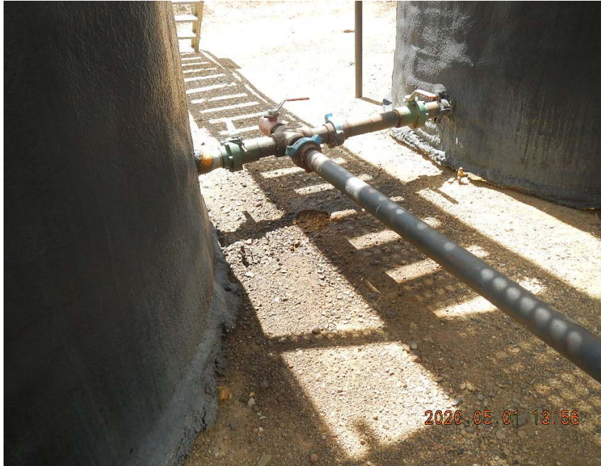
Tank 0030, staining beneath hammer unions.
