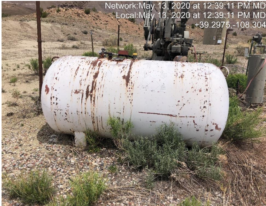
Photo #1179 Tank by wellhead is not properly labeled.
