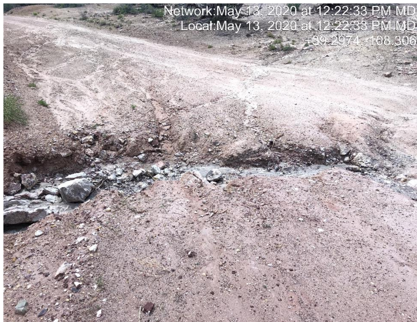
Photo #1173 Access road has not been adequately maintained.
