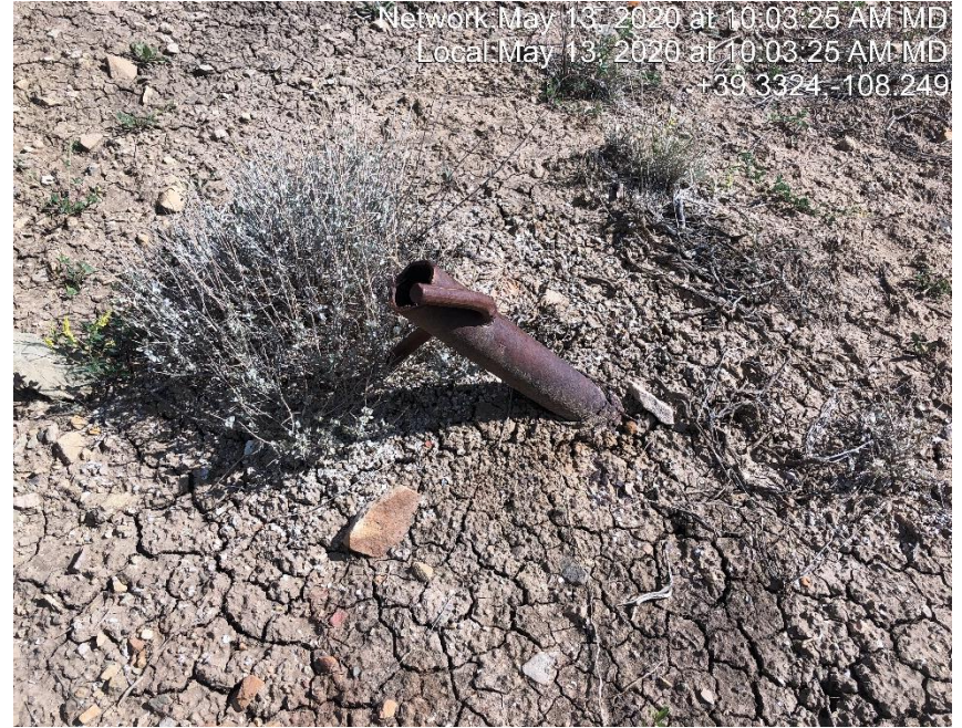
Photo #1168 Multiple unmarked deadman.
