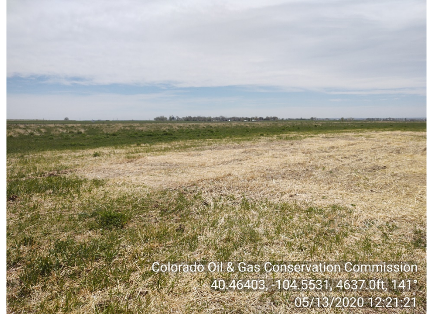
Photo #2 Ankeney 2-28 Battery site Abandoned: ALL Equipment removed Reclamation progressing
