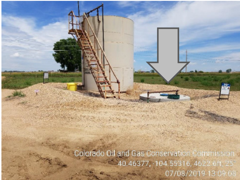
Photo #3 Ankeney 2-28 Battery site Inadequate berm height prior insp.
