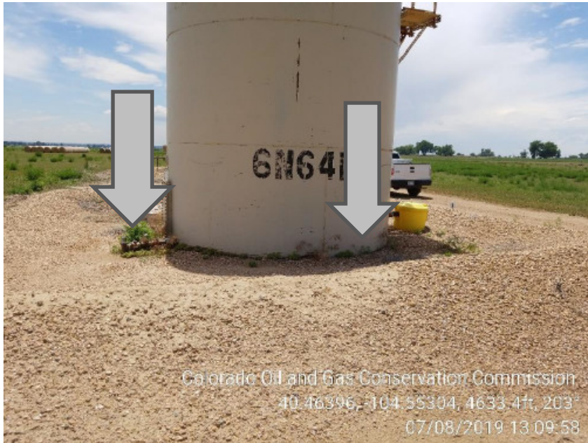
Photo #5 Ankeney 2-28 Battery site Weeds at tank site prior insp.
