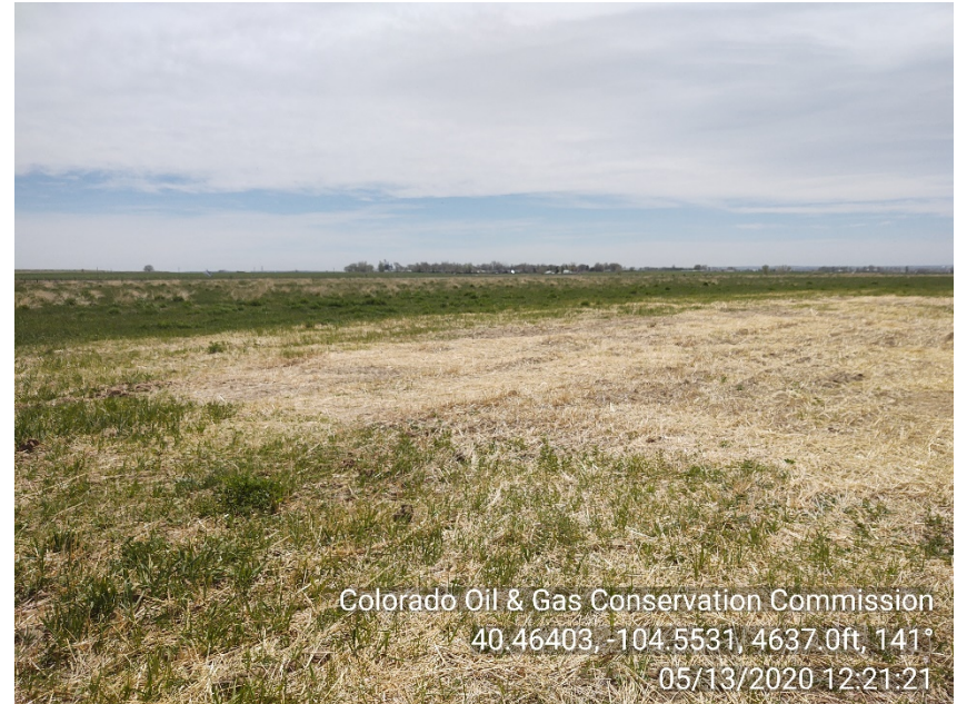
Photo #6 Ankeney 2-28 Battery site Abandoned: ALL Equipment removed Reclamation progressing Corrective Action mitigated
