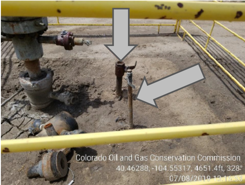
Photo #11 Ankeney 2-28 Wellsite Unmarked risers prior insp.
