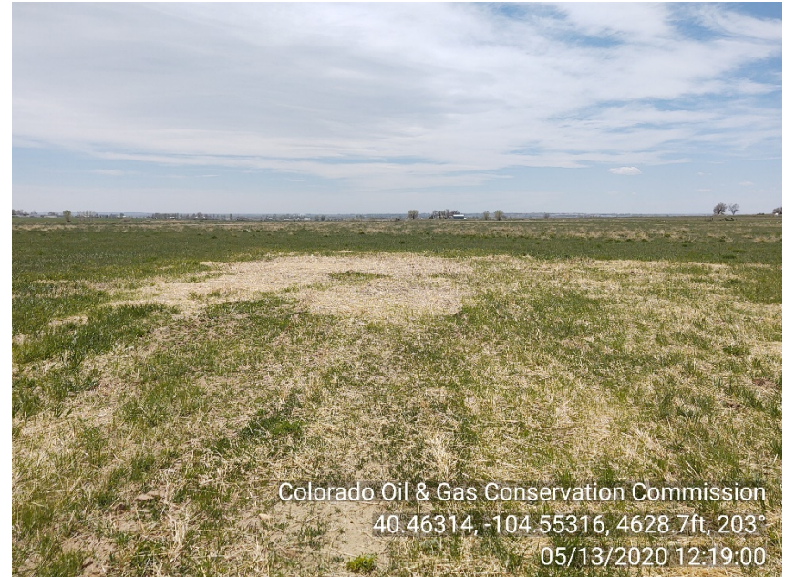
Photo #10 Ankeney 2-28 Wellsite Plugged & Abandoned | PA ALL Equipment removed Corrective Action mitigated
