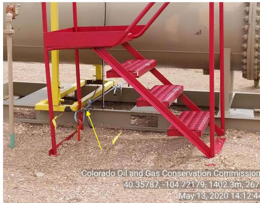
Photo 4: Separator anchored
