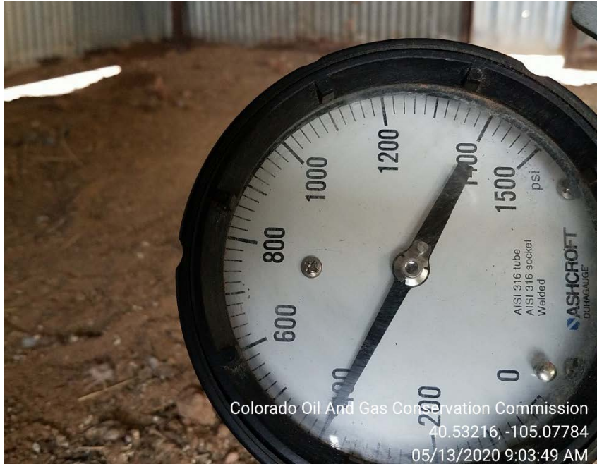
Starting casing test pressure
