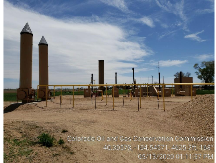
Photo #4 Separators, ECD's & Meter Runs
