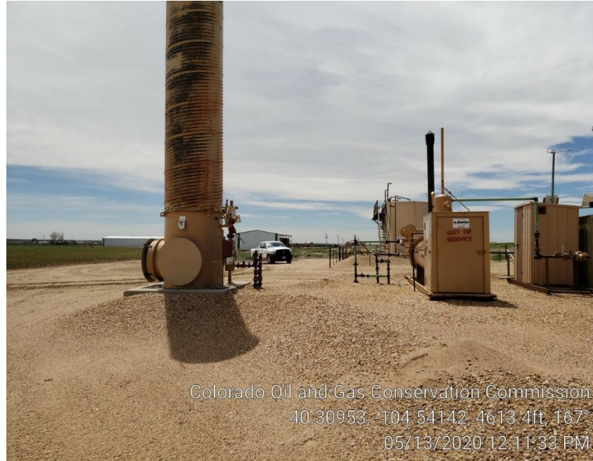
Photo #5 Separator, ECD & Meter Run
