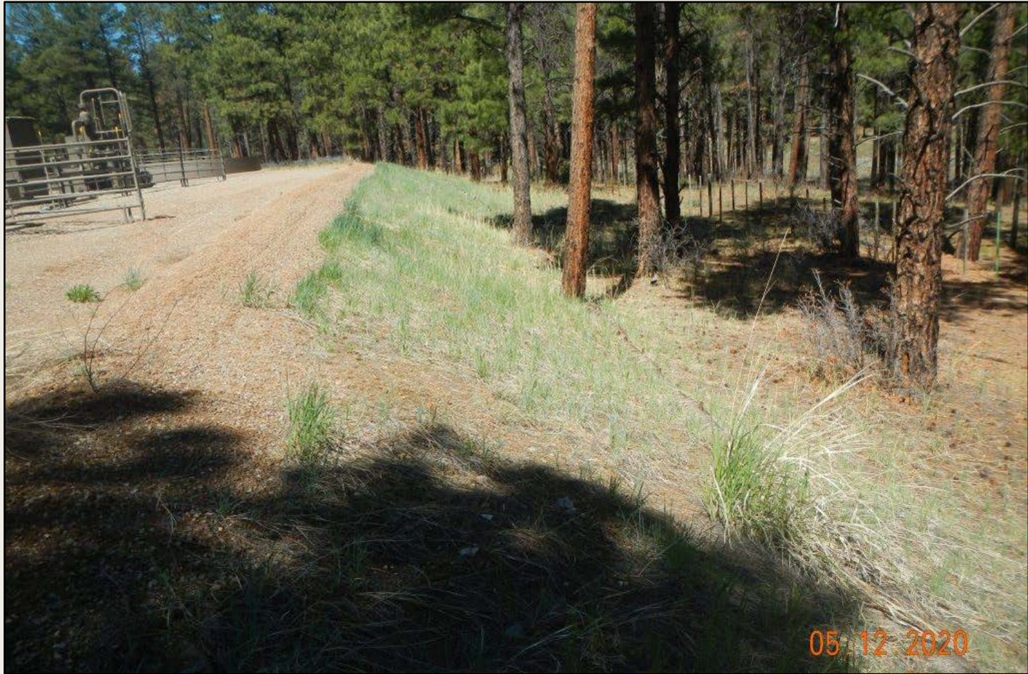
Photo 2. View of the northern fill slope from the northeastern corner facing westward. Revegetation is progressing with grasses such as smooth brome and western wheatgrass.
