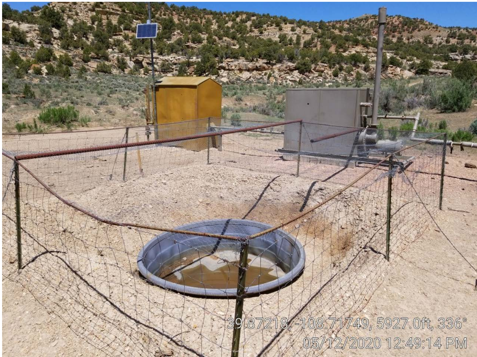
Photo 3. Tank, separator, and meter building.
