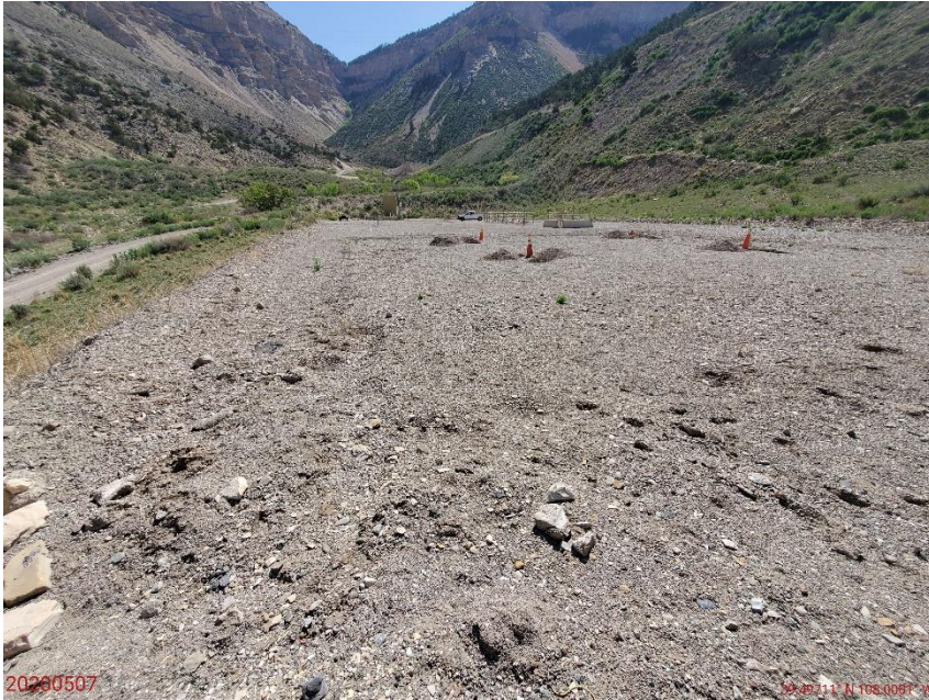
Photo 17: Photo taken from the northwest corner of the pad, facing east. Photo shows areas where a tank battery was Located. Facility has since been remove resulting in areas no longer needed for production subject to 1003 interim reclamation. Areas are being proposed for use by Operator to store drill cuttings from the NPR O04 Pad, to eventually be utilized for interim reclamation.
