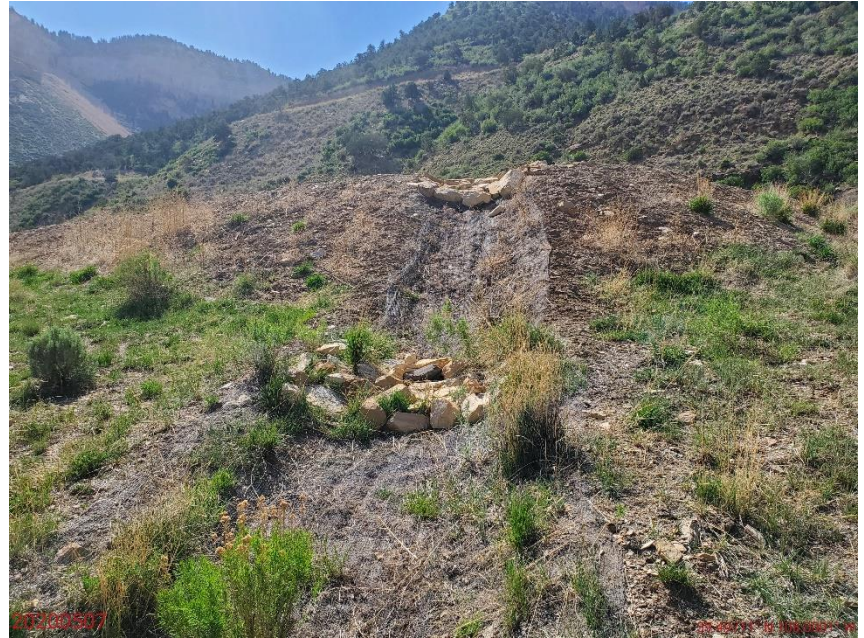
Photo 12: Photo taken from the northwest corner of the fill slope/pad. Photo shows rock checks and outlet.
