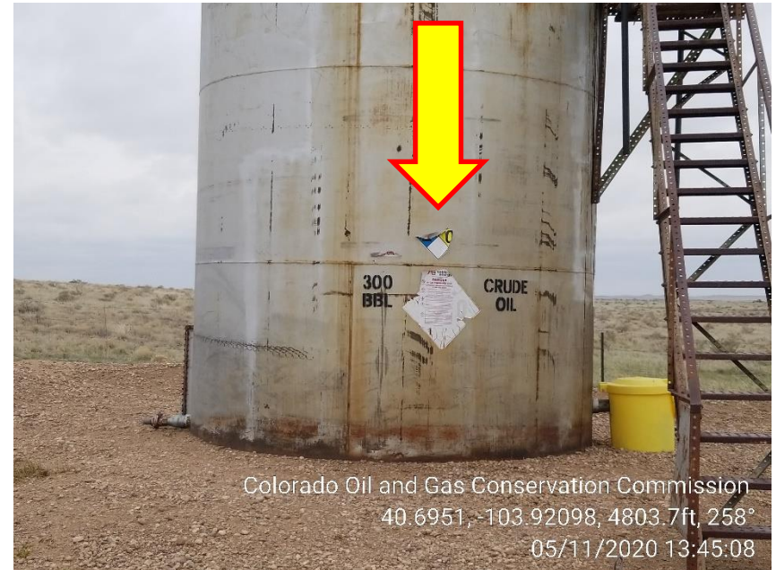
Photo 4 – NFPA Label has faded/peeled
