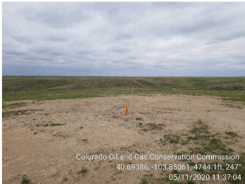
Photo 1 – Well PA'd; Cut and Capped
