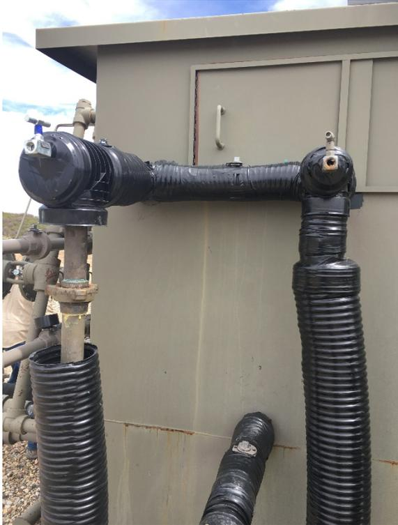
**Flowline failure was on produced water dump line. (left side) Wells are still producing. Operator has manifold at separator and is dumping produced water and oil into one dumpline and into one tank.**
