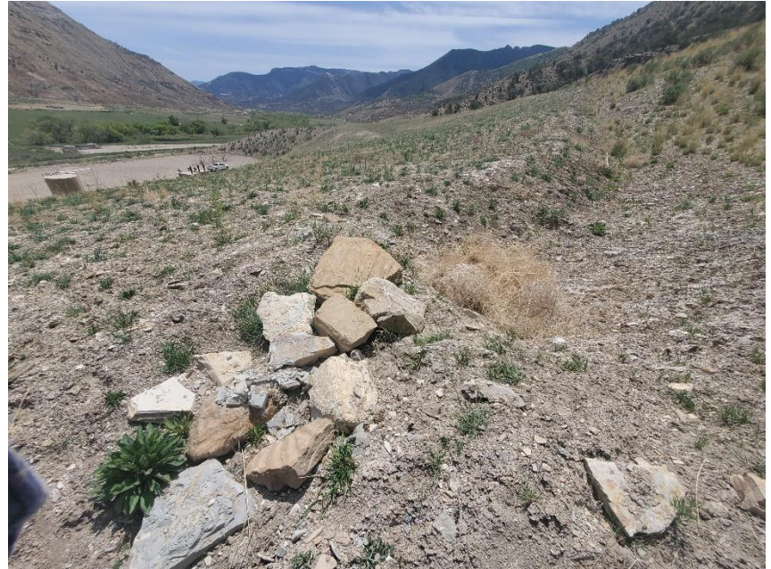
Photo 8: Photo taken from the northwest end of the Location, facing south. Photo shows sediment trap used in conjunction with ditch/berm.
