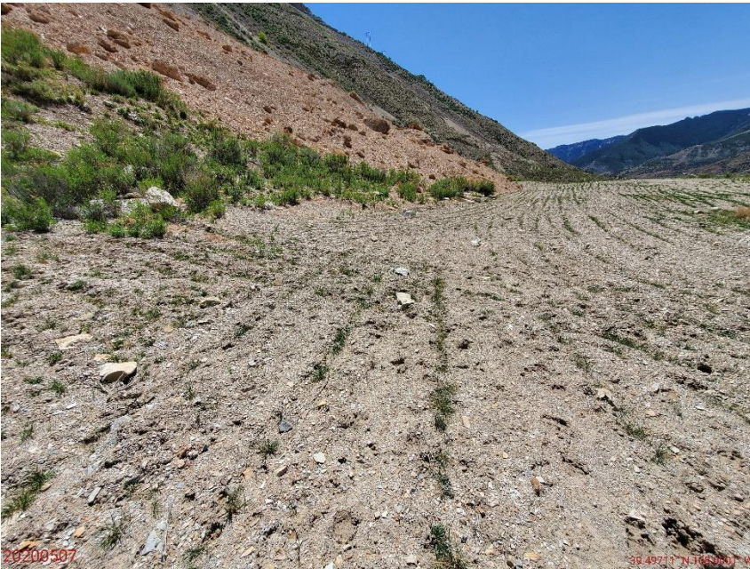
Photo 1: Photo taken from the north end of the Location, facing southeast. Photo shows Location remains flat, and has not been contoured in accordance with Rule 1004.a. Records indicate this is due to safety concerns regarding the stability of the adjacent landslide area.
