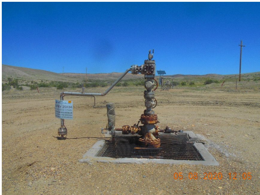
Injection wellhead
