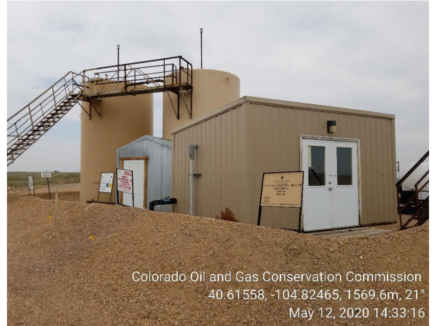
Photo 4: Produced water tanks
