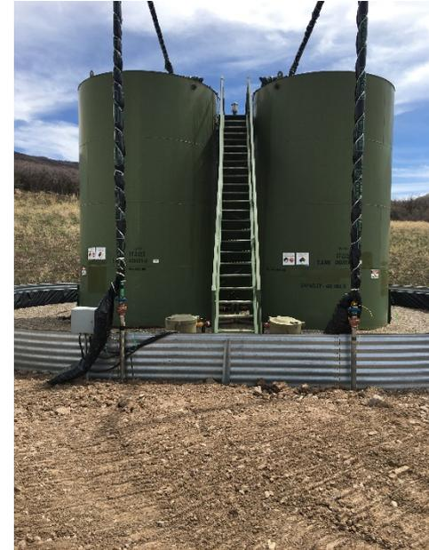
**New 2" stainless steel risers installed with tracer wire**
