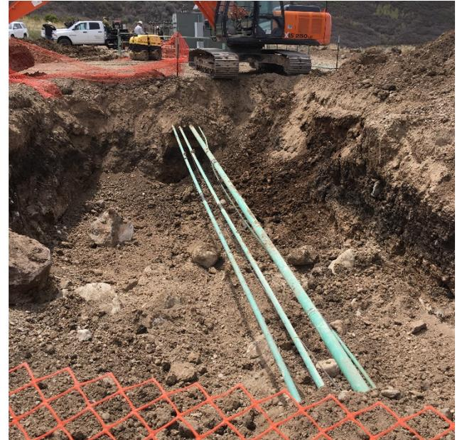
**Existing 2" carbon steel Flowlines was taken out of service and will be plugged and abandoned when location is reclaimed. Flowline was capped and cut 3' under dirt grade**
