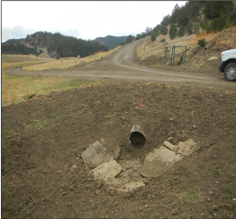
Photo 1. The culvert along the main road has been repaired however, the culvert is filled in with sediment which will create issues.
