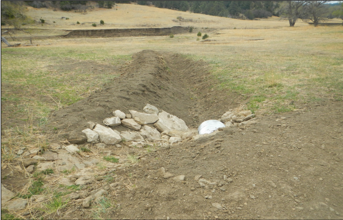
Photo 1. The culvert outlet has been repaired. Additional outlet protection may be needed to prevent erosion of the diversion ditch.
