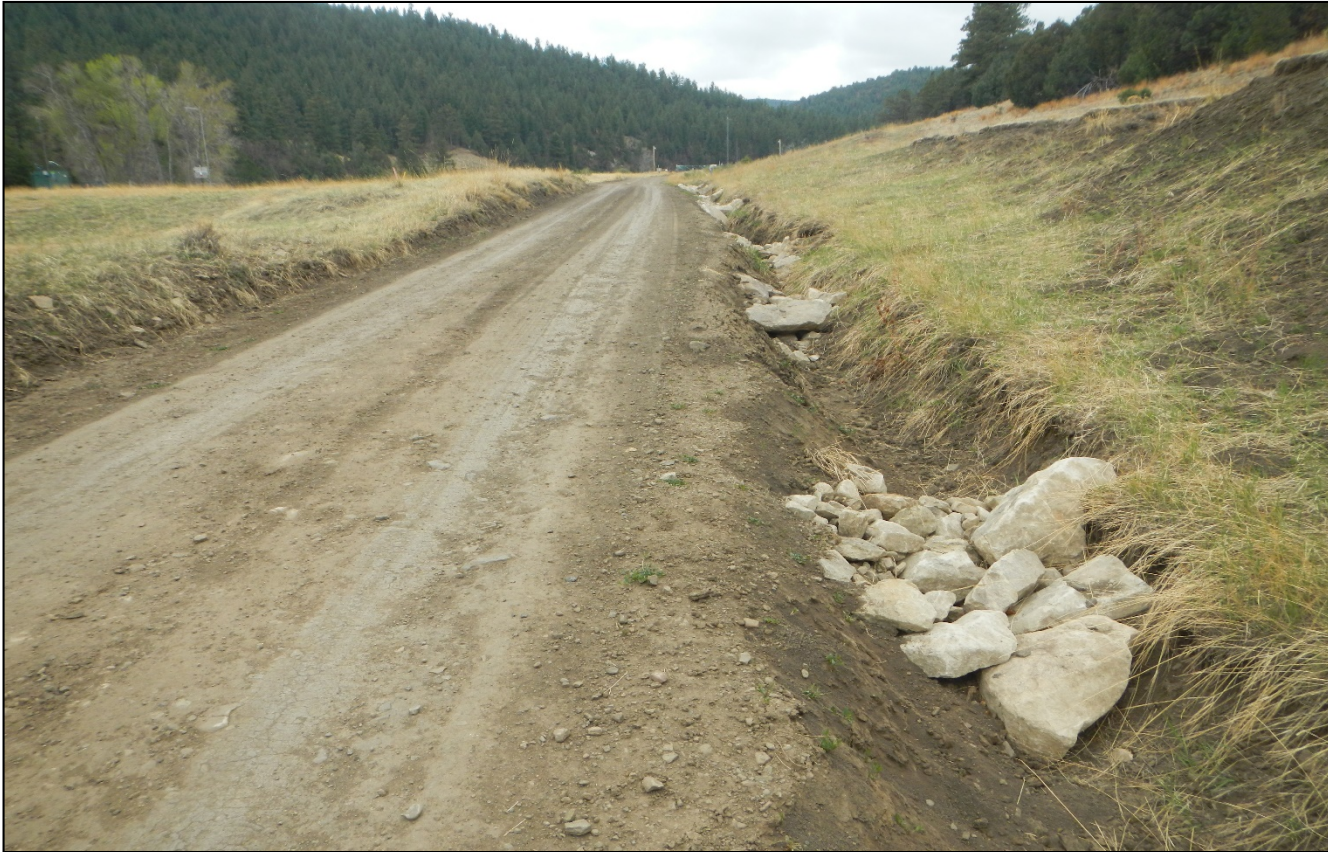
Photo 4. Rock check dams have been installed along the side of the road where erosion occurred. This will need to be monitored to ensure stormwater does not flow around the check dams causing further erosion.
