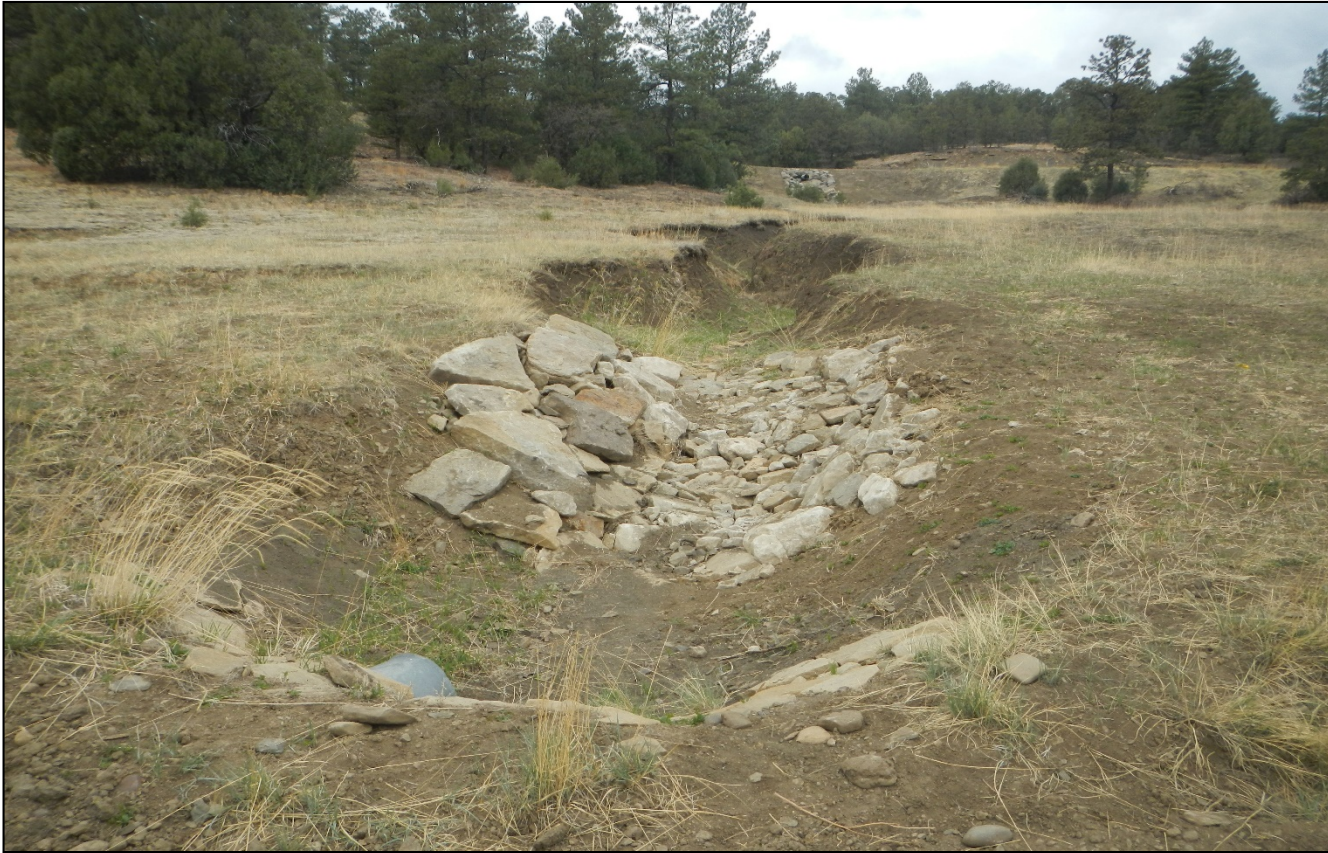
Photo 2. Facing toward the culvert inlet. Additional culvert inlet protection was installed. Disturbance areas caused by erosion may need to be reclaimed.
