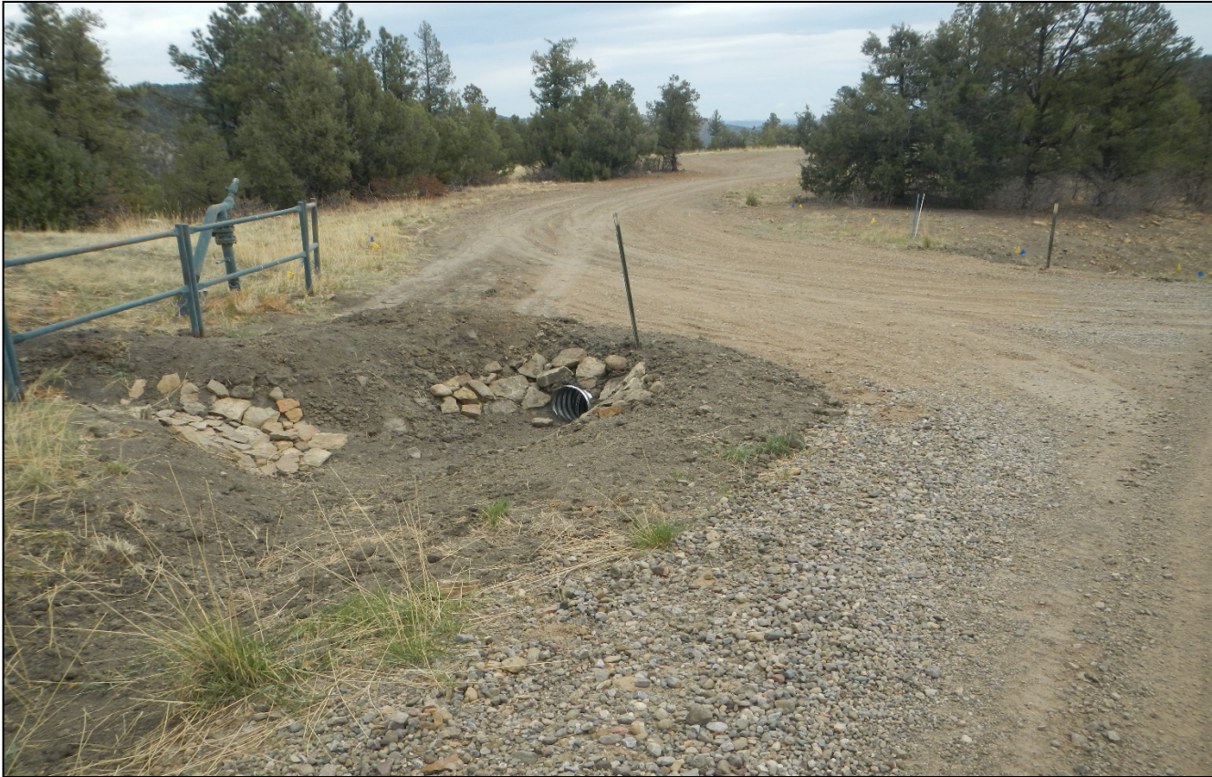
Photo 1. The culvert at the beginning of the access road has been repaired.
