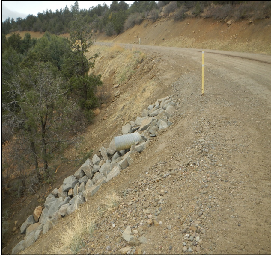
Photo 7. Further up the main road toward the location. The culvert inlet has been maintained and sediment removed. Outlet protection has been installed at culvert outlet where erosion was previously observed.
