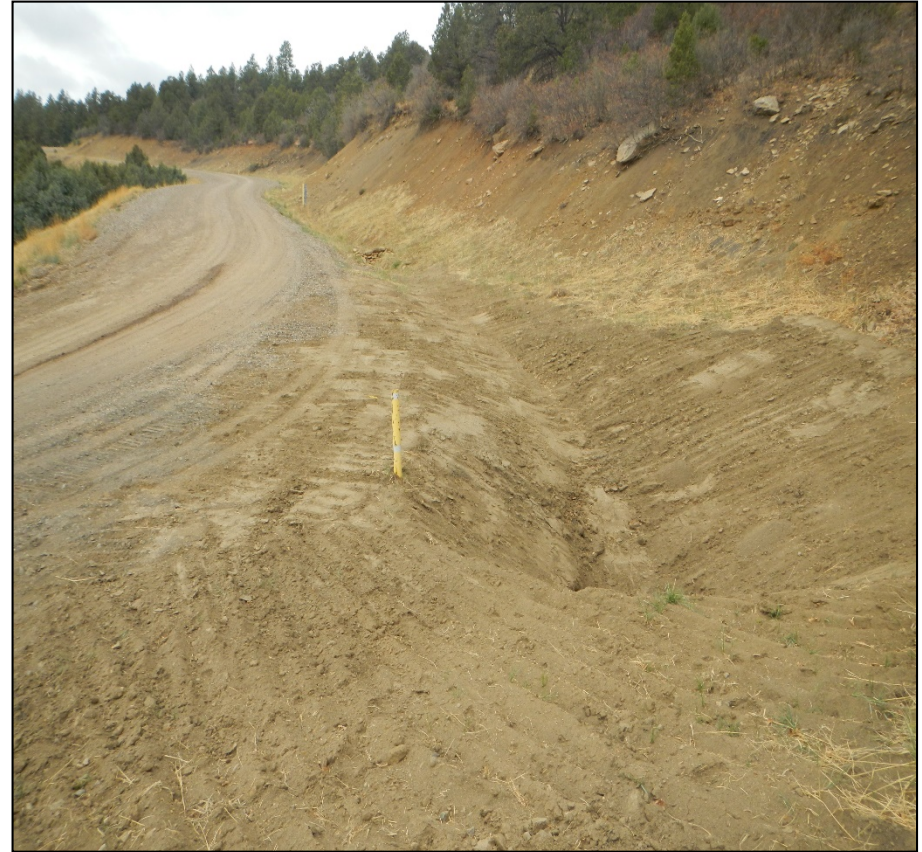
Photo 7. Further up the main road toward the location. The culvert inlet has been maintained and sediment removed. Outlet protection has been installed at culvert outlet where erosion was previously observed.
