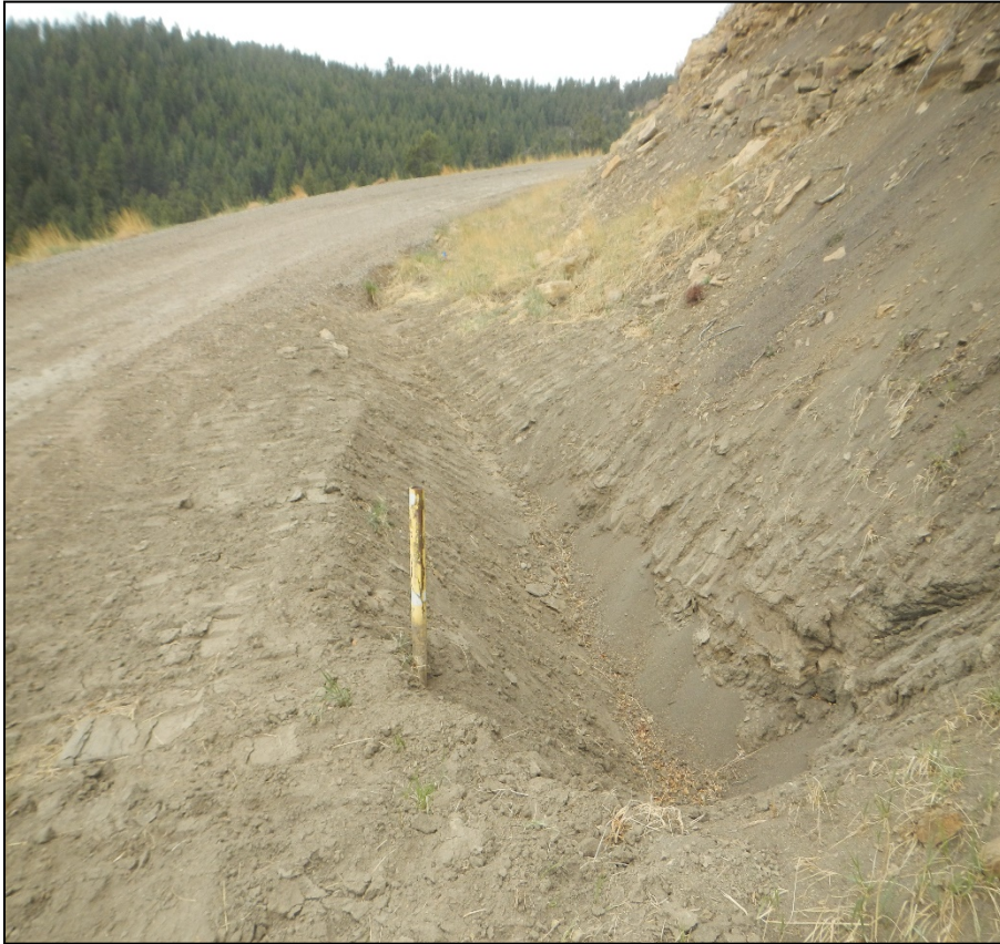
Photo 6. The culvert inlet has been maintained and sediment removed. Outlet protection has been installed at culvert outlet where erosion was previously observed.
