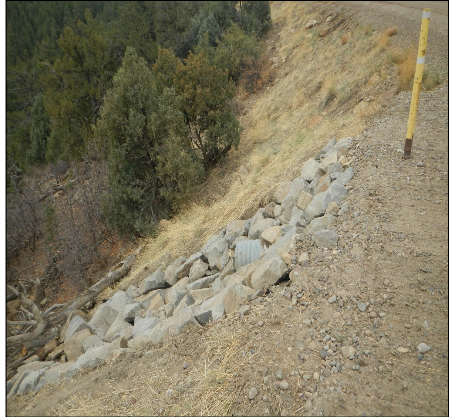
Photo 6. The culvert inlet has been maintained and sediment removed. Outlet protection has been installed at culvert outlet where erosion was previously observed.
