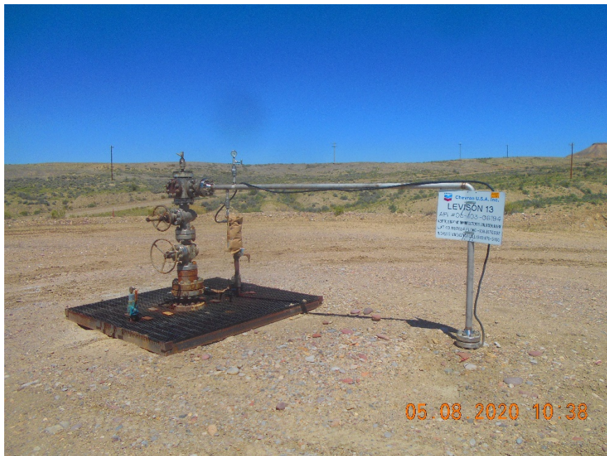
Injection wellhead
