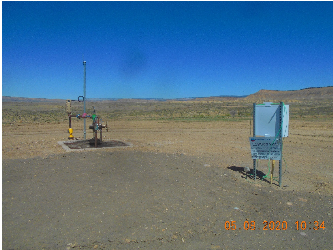
Injection wellhead – Converted to Producer
