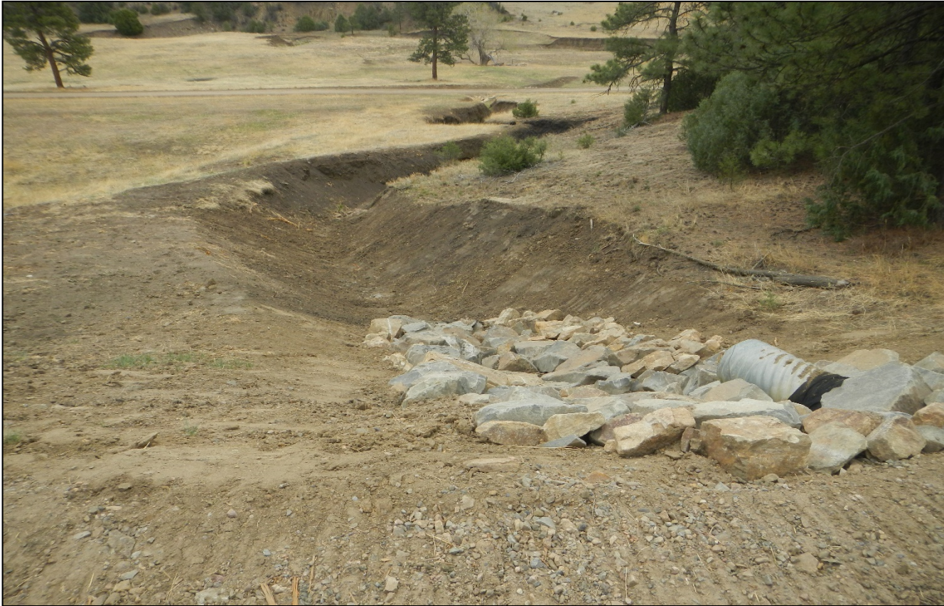
Photo 1. Outlet protection has been installed at the culvert. It appears stormwater from the road has been directed to this area causing this erosion gully. Disturbance areas caused by erosion may need to be reclaimed.
