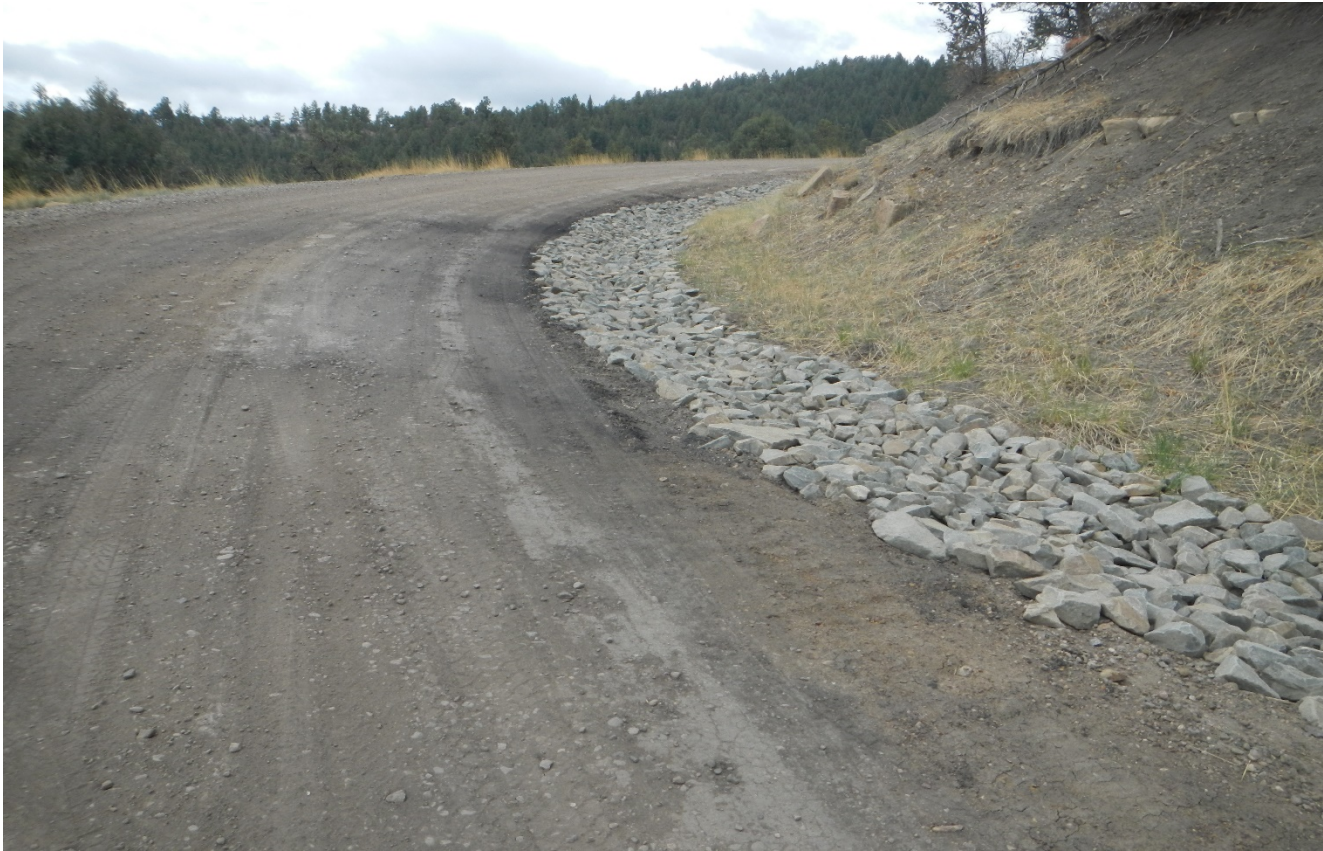
Photo 5. Further up the main road. Rock rip/rap has been installed along the side of the road to prevent erosion.
