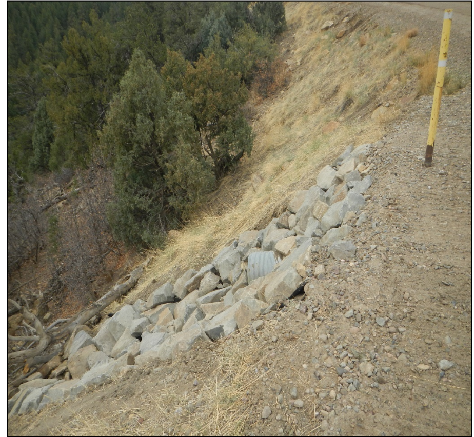
Photo 6. The culvert inlet has been maintained and sediment removed. Outlet protection has been installed at culvert outlet where erosion was previously observed.
