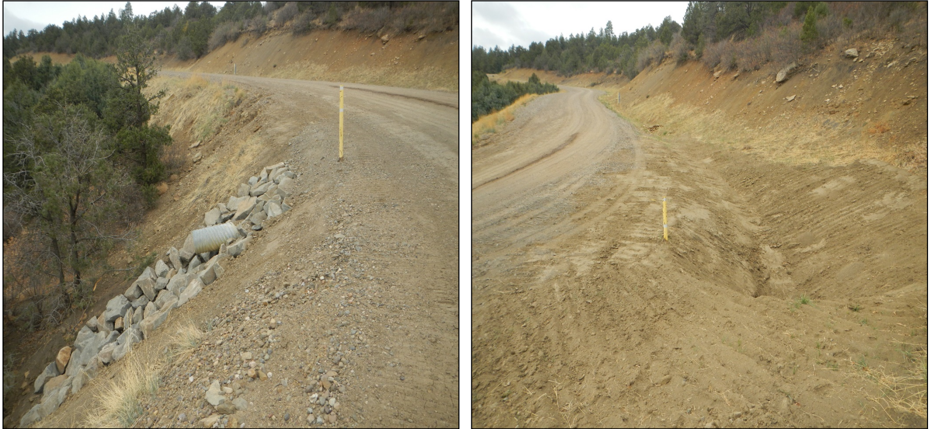
Photo 7. Further up the main road toward the location. The culvert inlet has been maintained and sediment removed. Outlet protection has been installed at culvert outlet where erosion was previously observed.
