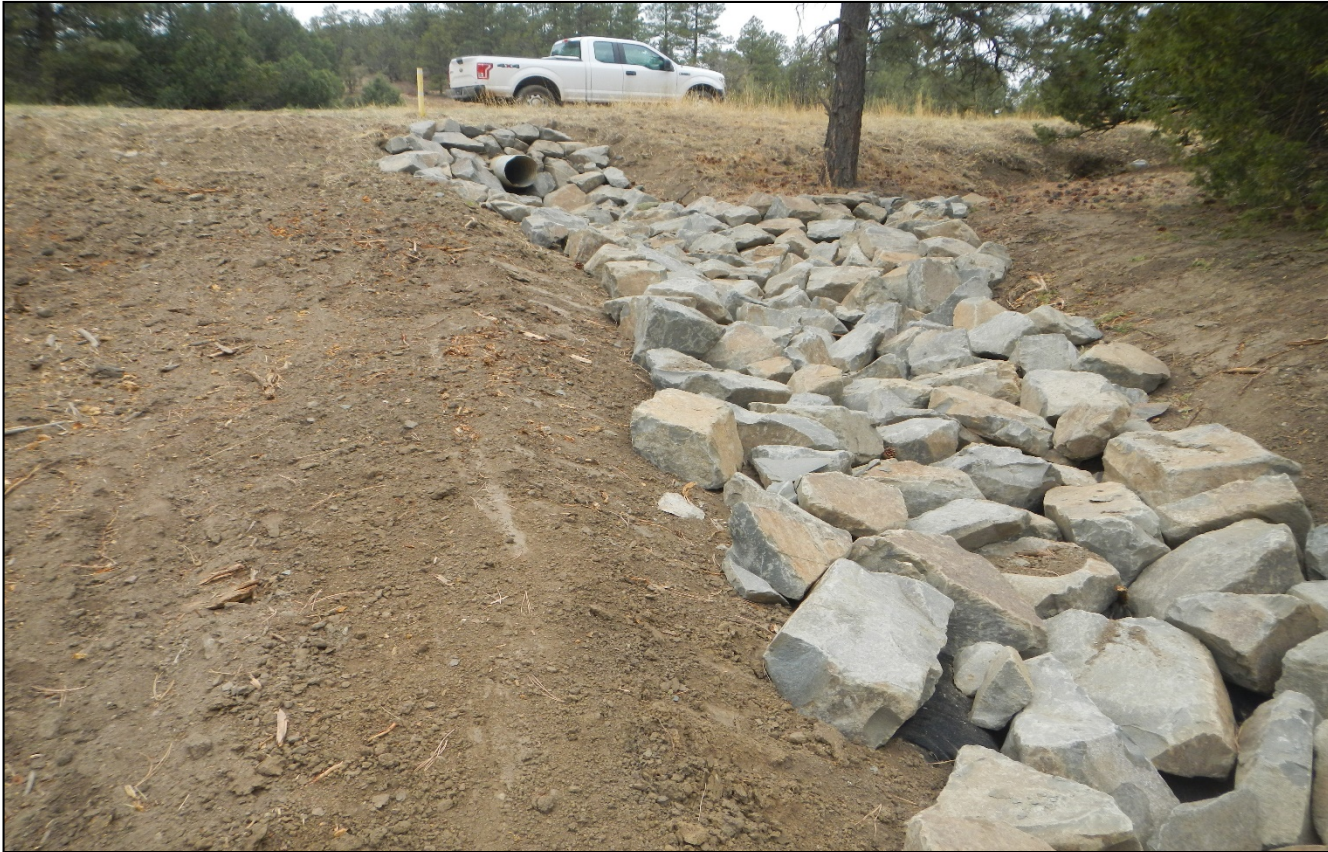
Photo 2. Further up the road, outlet protection has been installed where erosion was during previous inspection.
