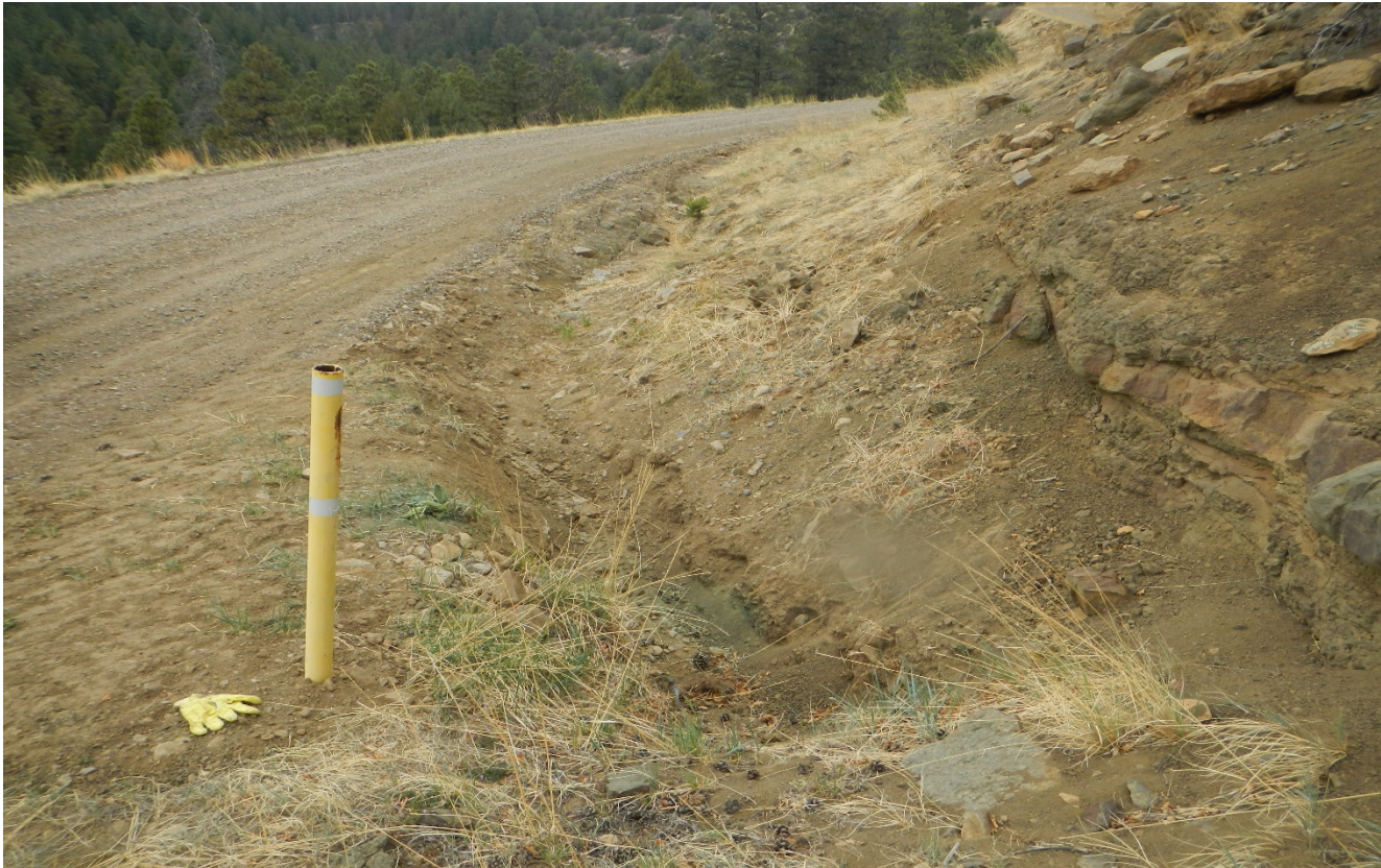
Photo 10. The culvert inlet has been cleaned out of sediment and maintained.
