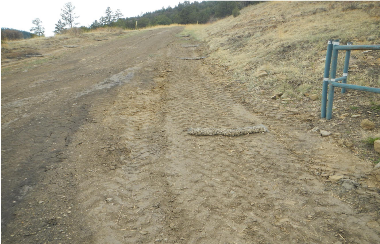
Photo 7. Rock wattles have been placed on the side of the access road. It is uncertain if the rock wattles will withstand the stormwater flow. These will need to be monitored and maintained to ensure stormwater does not displace or flow around.
