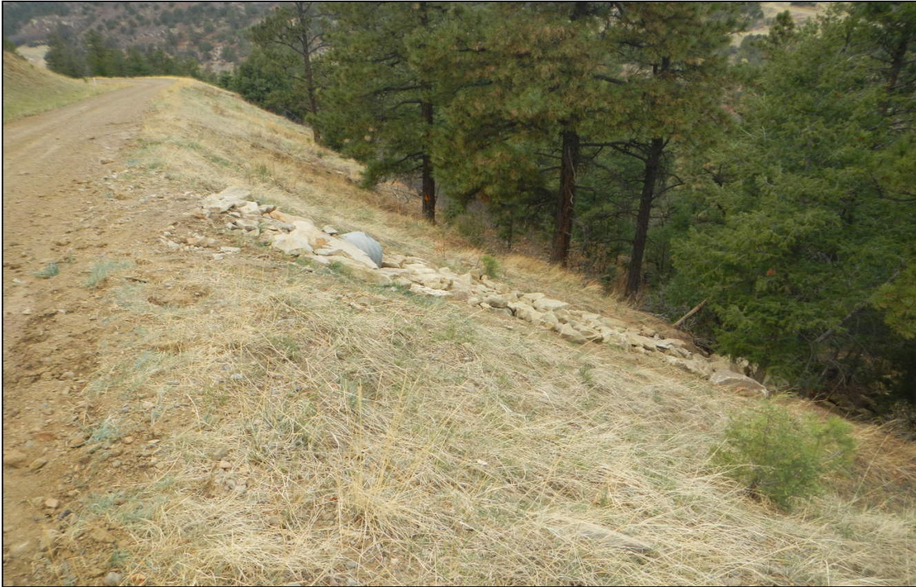
Photo 2. Culvert outlet protection has been installed at the culvert where erosion was observed.
