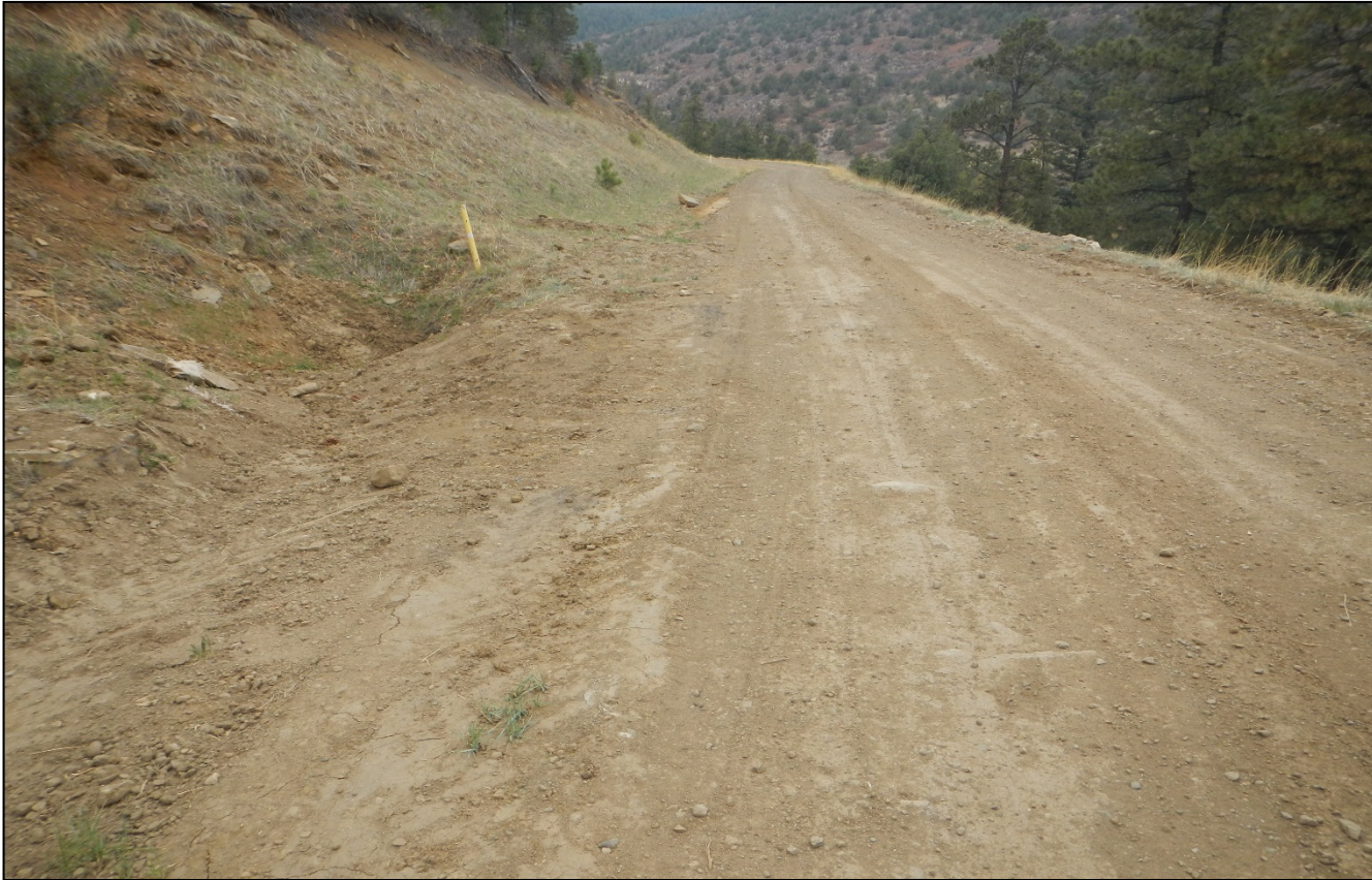
Photo 1. There erosion near culvert inlet has been repaired.
