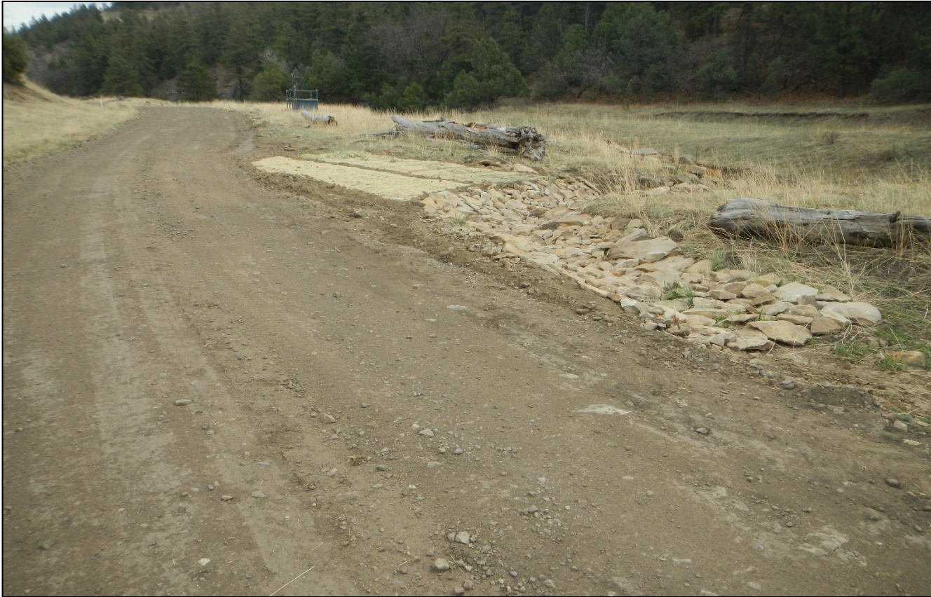
Photo 4. Culvert outlet protection has been installed at the culvert where erosion was previously observed.
