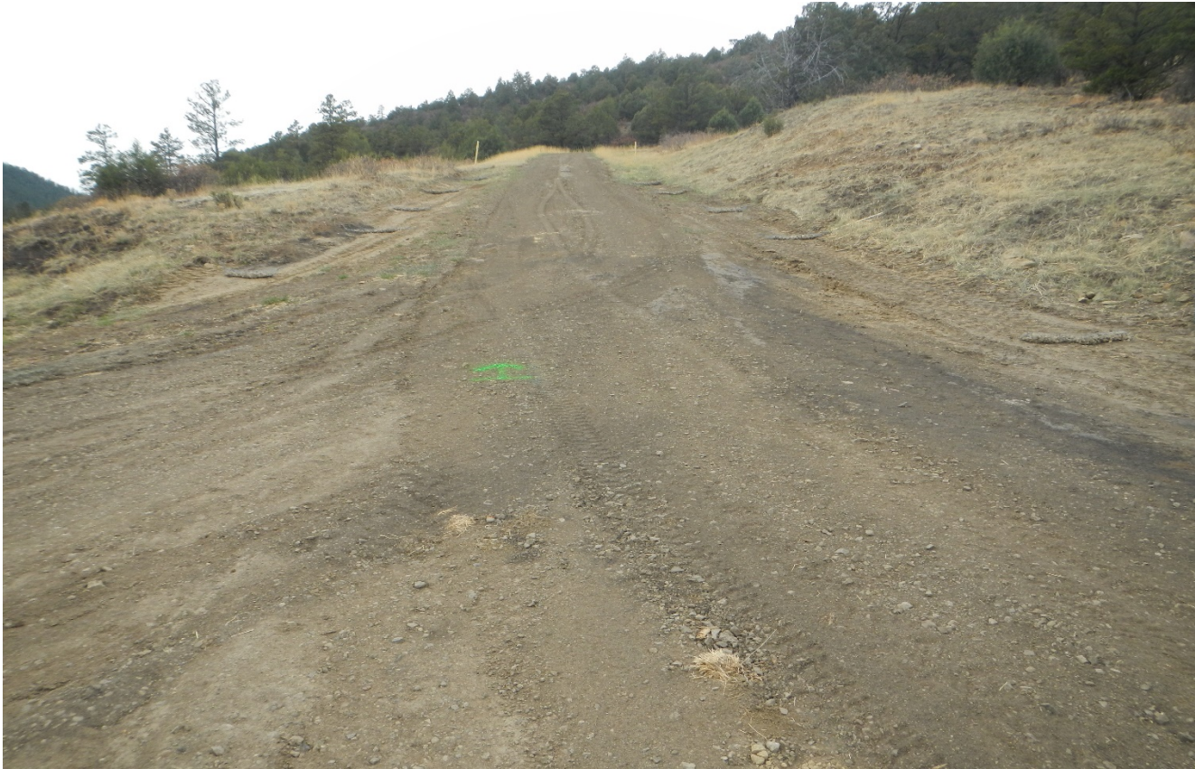
Photo 6. Facing toward the access road. The erosion along the sides of the access road have been repaired.
