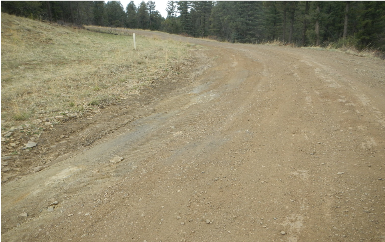
Photo 9. The area of erosion along the road has been graded and repaired.
