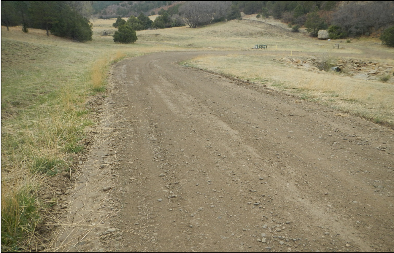
Photo 3. The road has been graded where erosion was previously occurring.
