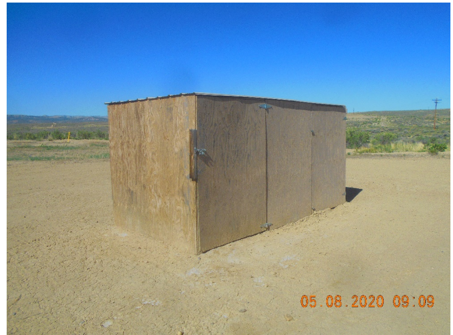
Injection wellhead housing
