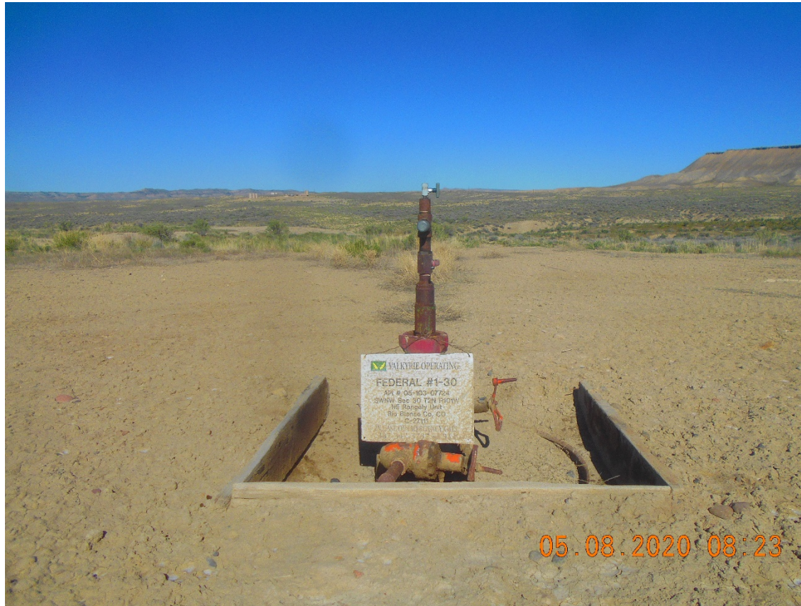
Injection Wellhead – Temporarily Abandoned
