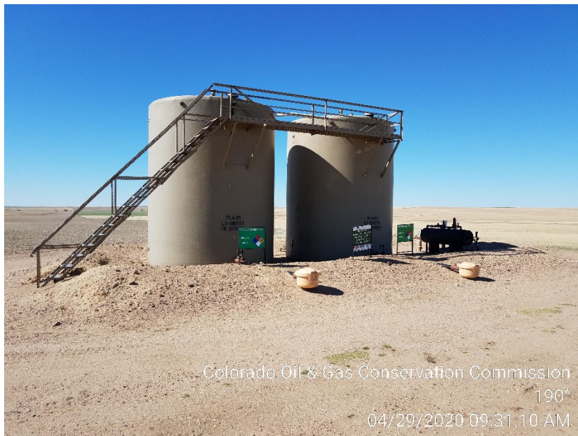
3. Tank battery , Free Water Knockout.
