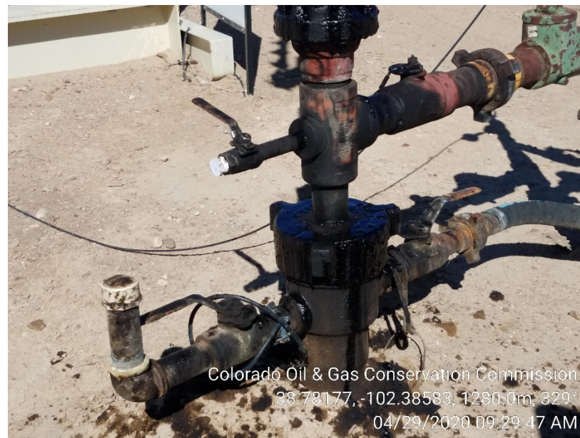
4. Casing open and venting to atmosphere.
