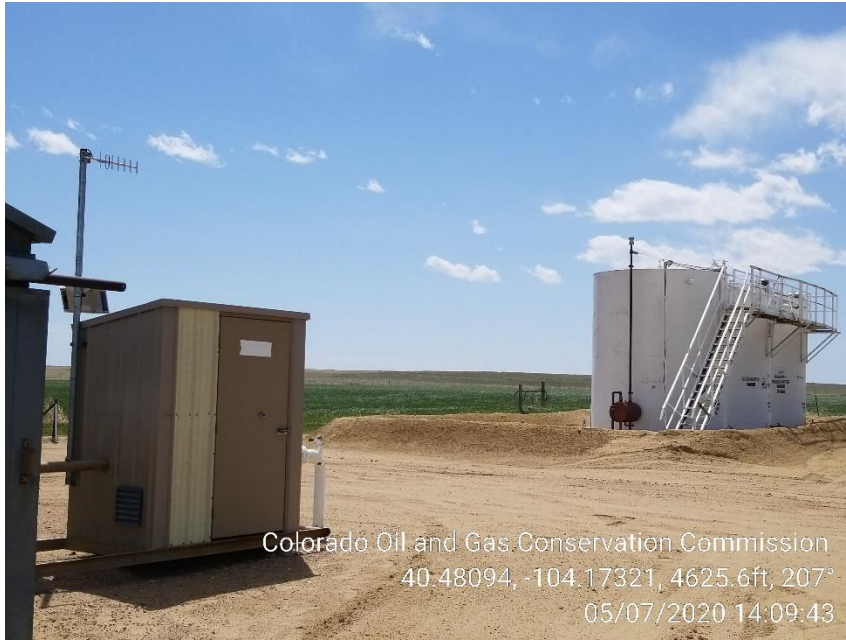
Photo 3 – Tank Battery
