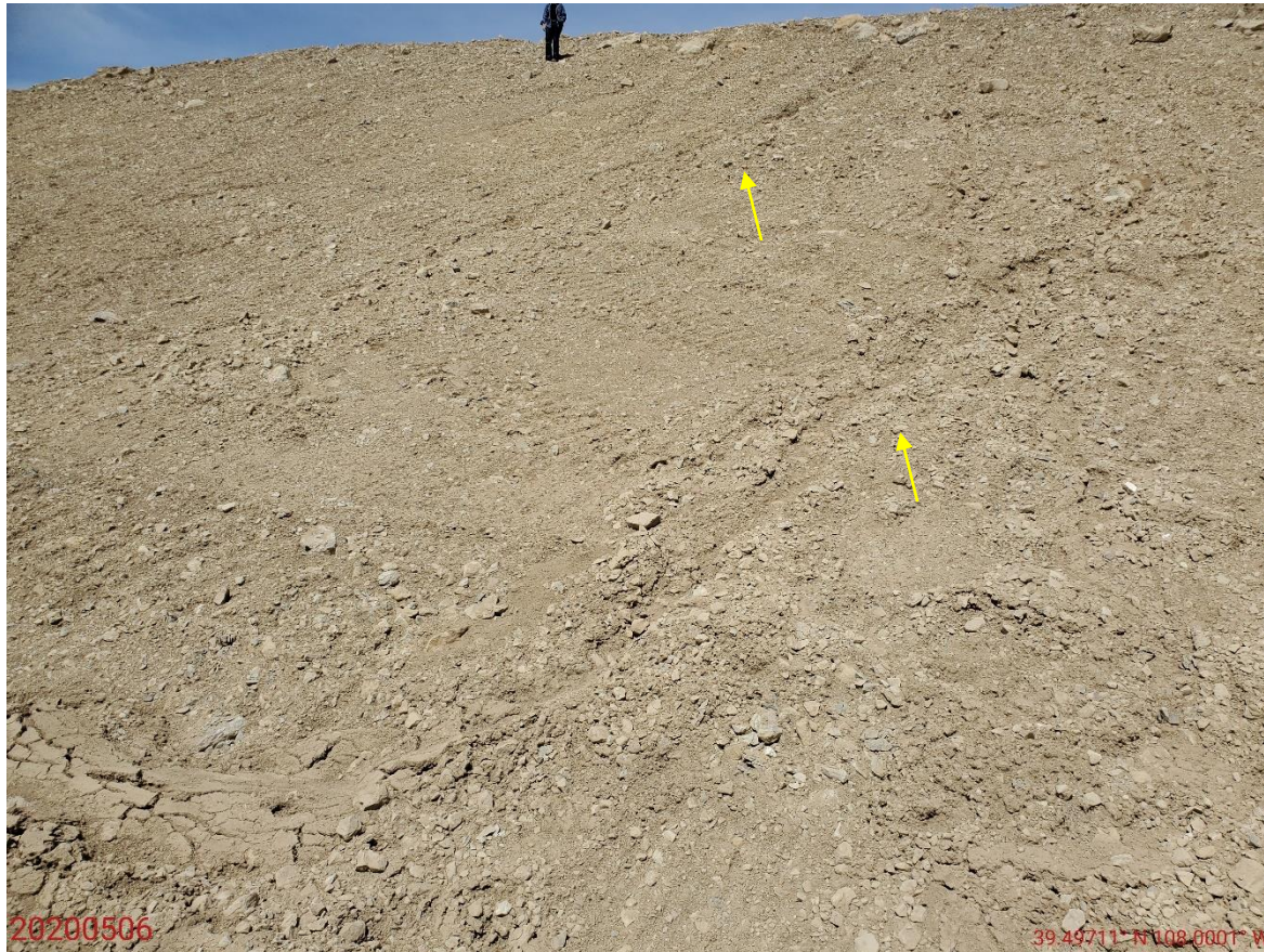
Photo 8: Continued from photo 7. Photo shows areas where rill erosion/erosion degradation on the slopes of the Location is evident; BMPs remain missing or insufficient. Photo also shows interim reclamation (revegetation activities) has not been completed. Inspector at top of photo for reference.
