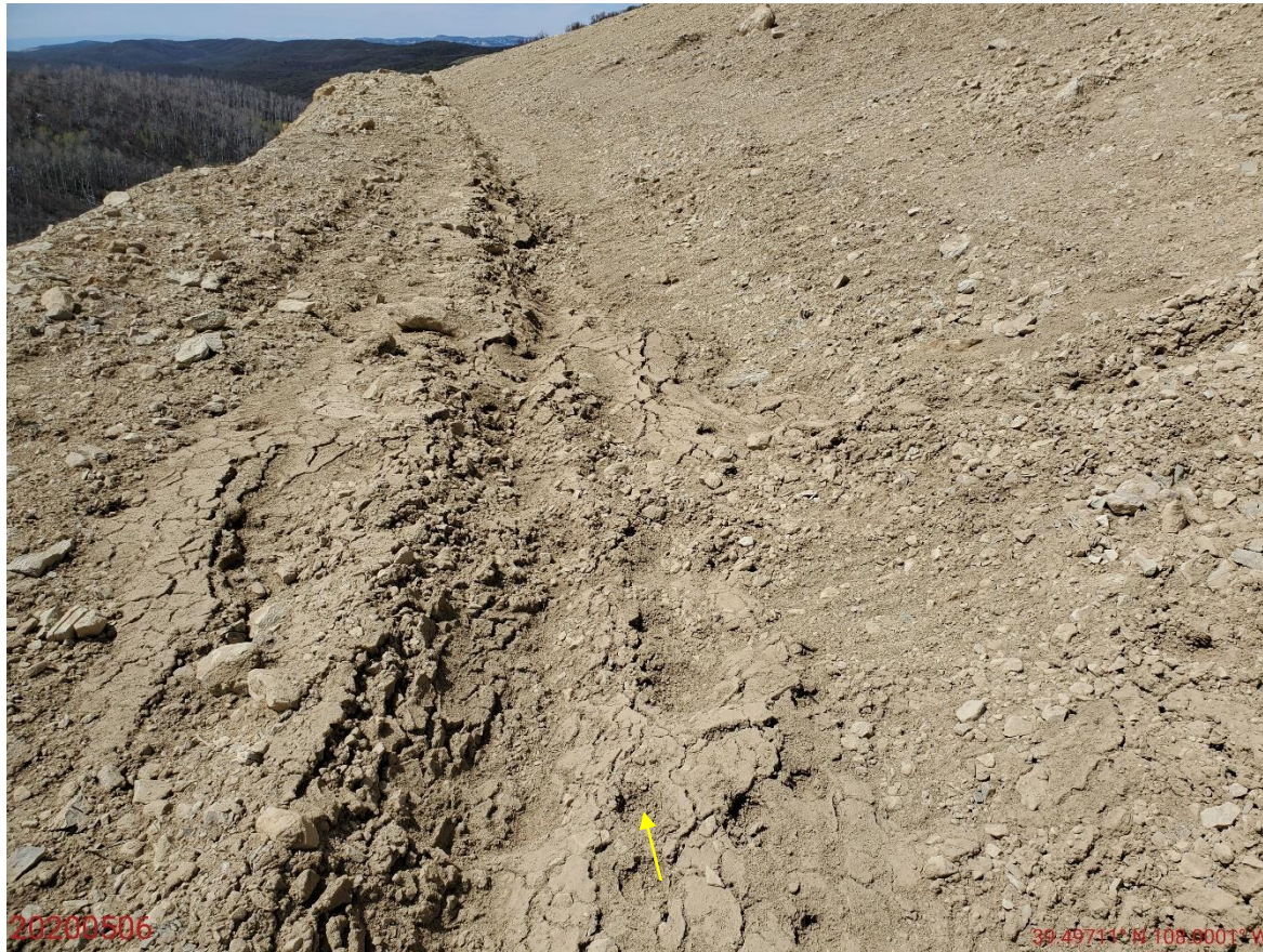
Photo 9: Continued from photo 8. Photo shows sediment deposition due to erosion from the slopes.
