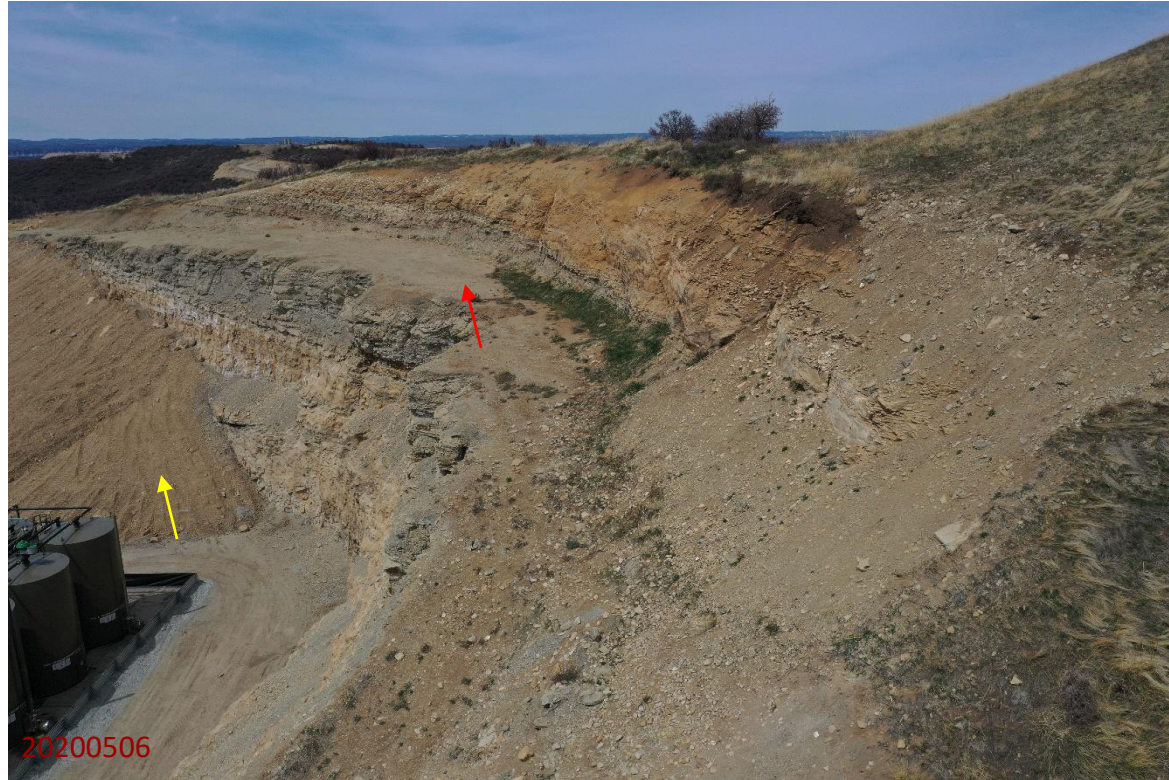
Photo 6: Continued from photo 5. Photo shows areas on the northern end of the Location where soil replacement/contouring has been conducted (yellow). Photo also shows areas on the northern end of the Location that have not been contoured (red). Photo also shows interim areas where BMPs appear to be missing, or insufficient, and where interim reclamation (revegetation activities) has not been completed.
