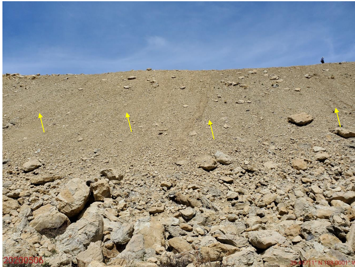
Photo 7: Photo taken from the southeast end of the Location, facing northwest. Photo shows areas where rill erosion/erosion degradation on the southeastern slopes of the Location is evident; BMPs remain missing or insufficient. Photo also shows interim reclamation (revegetation activities) has not been completed. Inspector at top right of photo for reference.
