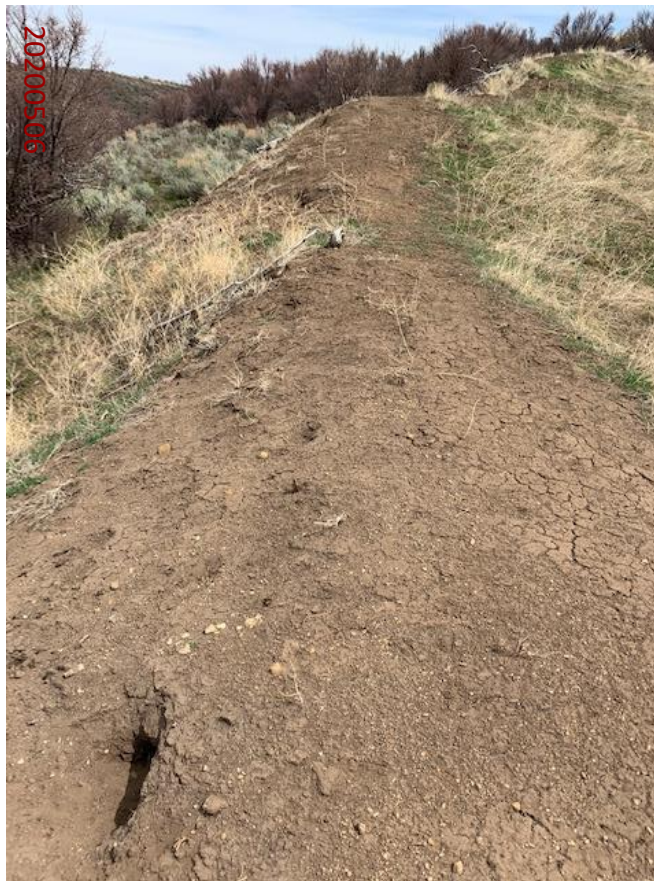
Photo 14: Photo taken from the topsoil stockpile on the northwest end of the Location. Photo shows soil stockpile is predominantly exposed soil, or vegetated by undesirable weedy plant species.
