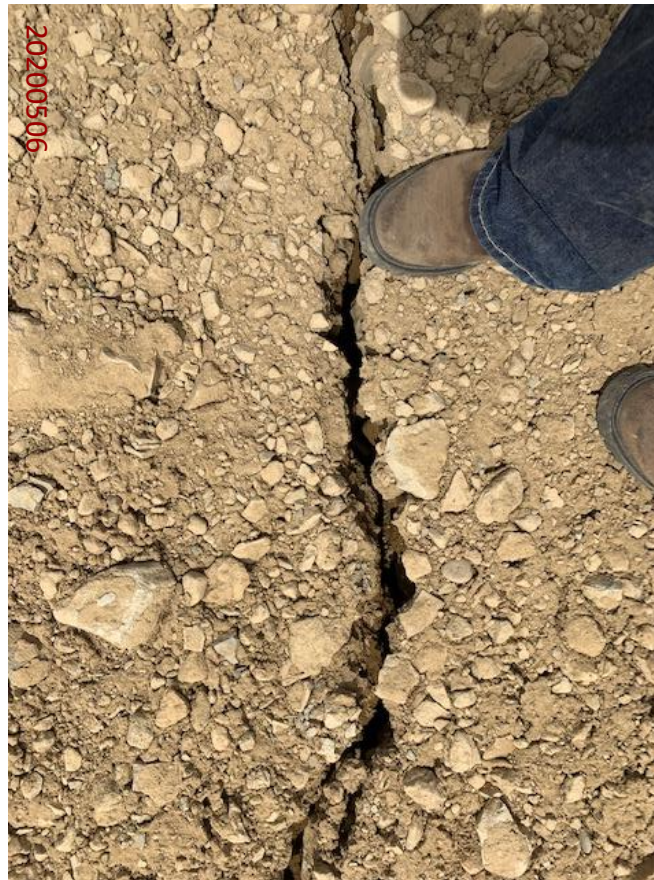
Photo 12: Photo taken from the slopes on the north end of the Location. Photo shows a crack forming along the interim areas indicating soils are unstabilized and are beginning to shift/slough.
