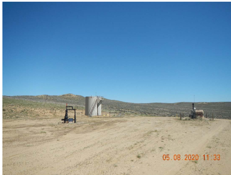
Photo 1. Overview of location taken facing north.
