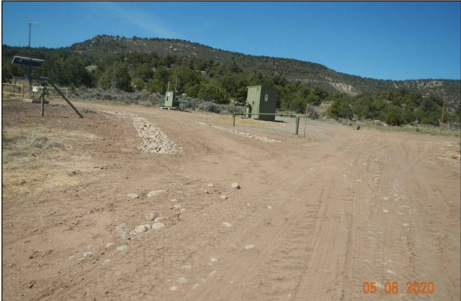
Photo 1. View of the southern project area from the well pad entrance facing center. Erosional channels are lined with rock, Russian thistle debris is removed.
