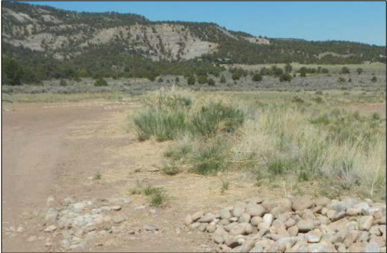
Photo 3. View of the central fill slope facing westward. Cobble lined rundowns placed in erosional features.
